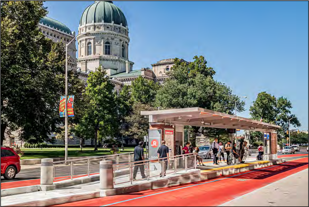
Example Photo: Existing Red Line Statehouse Station
