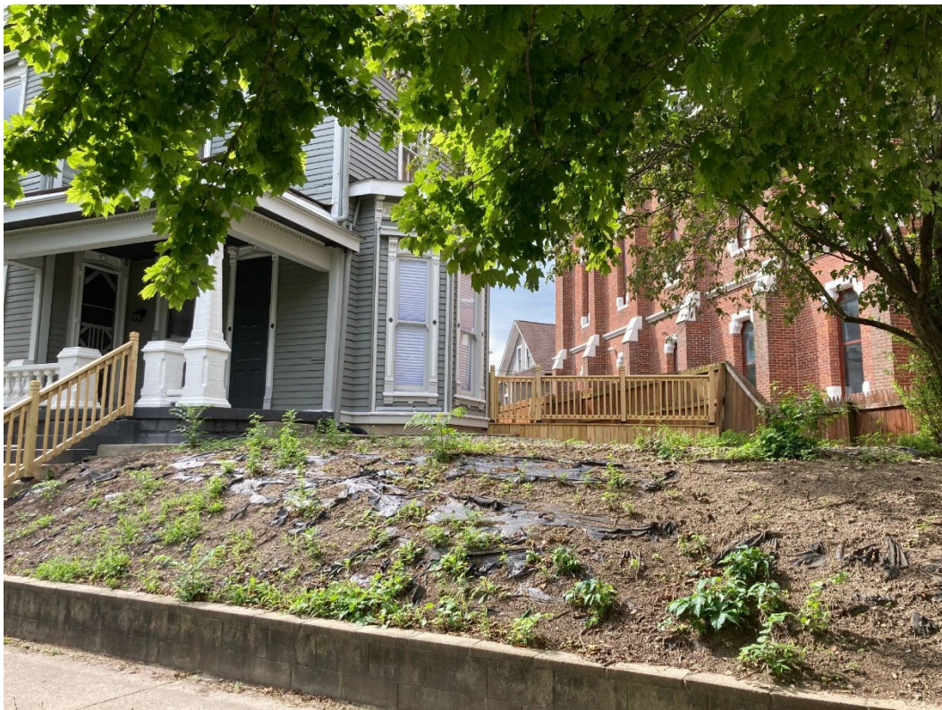
July 2021. Deck before fence installation.
