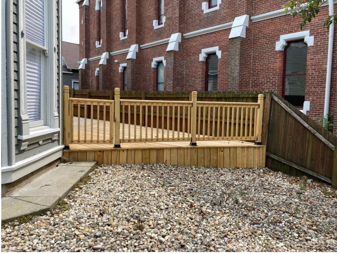
July 2021. Deck before fence installation.
