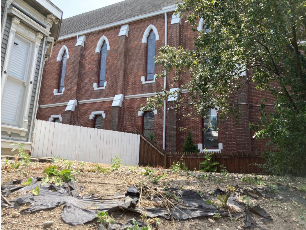
June 2023. Deck located behind white fence.
