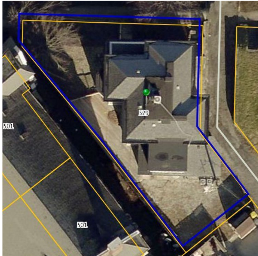
Nov 2021 – Jan 2022 aerial photo after deck extension.
