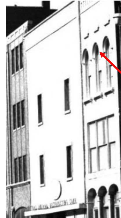
1978: Combined 231, 235 Source: National Register of Historic Places; 48 years, probably longer
