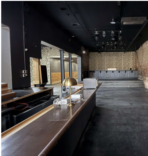
H: View of former stage. Demising wall seen on left side.
