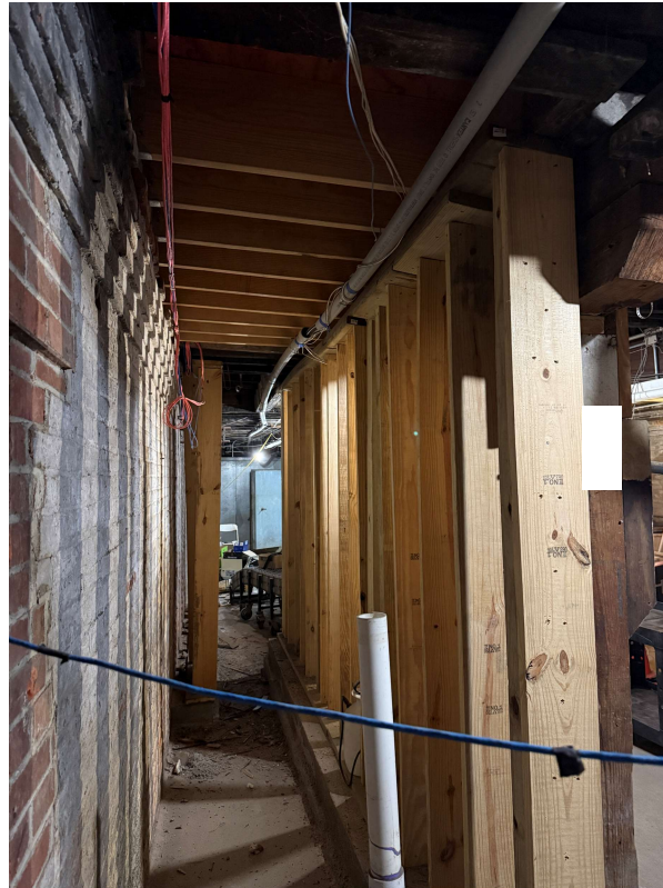
E: Additional supports added to carry weight of floor above
