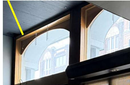
Arches on right side of 231 are in front of storefront windows
