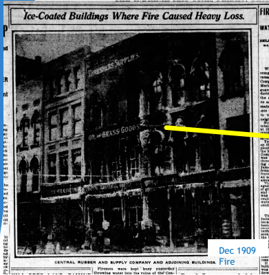
229 & 231: 1909 fire heavily damaged all floors
