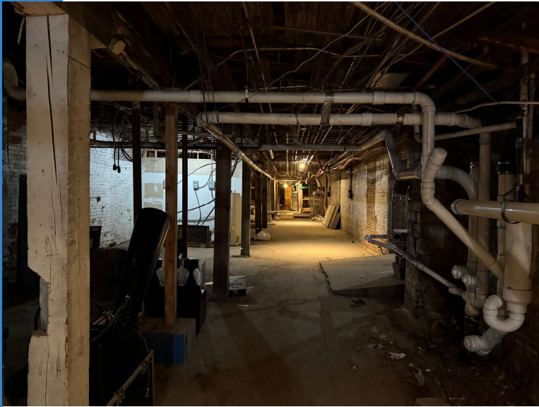
D: Basement area. Not usable. Primarily plumbing and storage. Low clearance.
