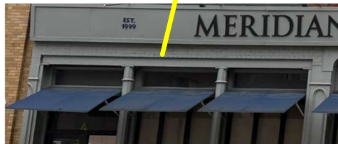
231: Arched windows removed & replaced with steel beam
