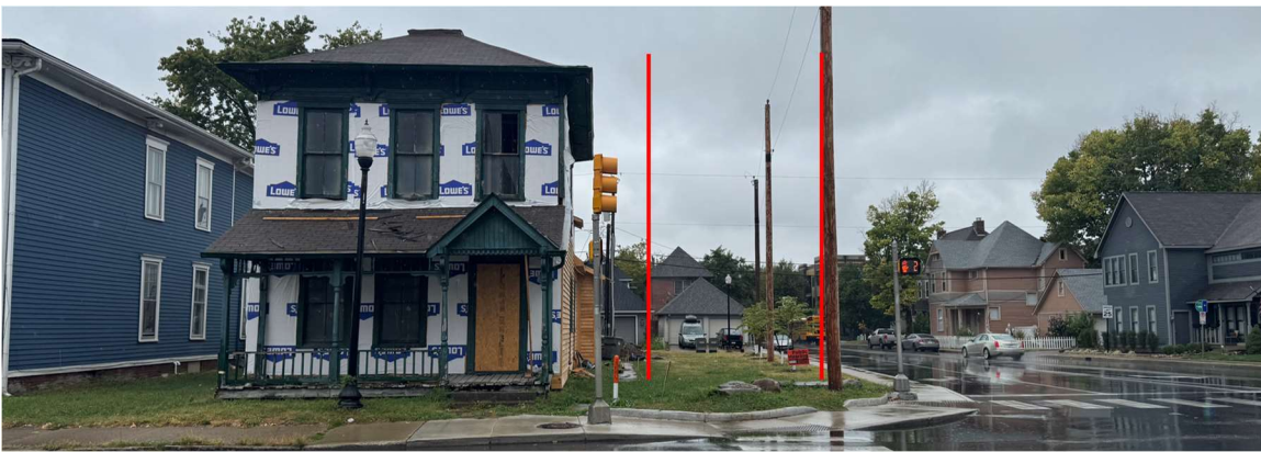
Red lines highlighting on site stakes to show width of the house's front façade as proposed
