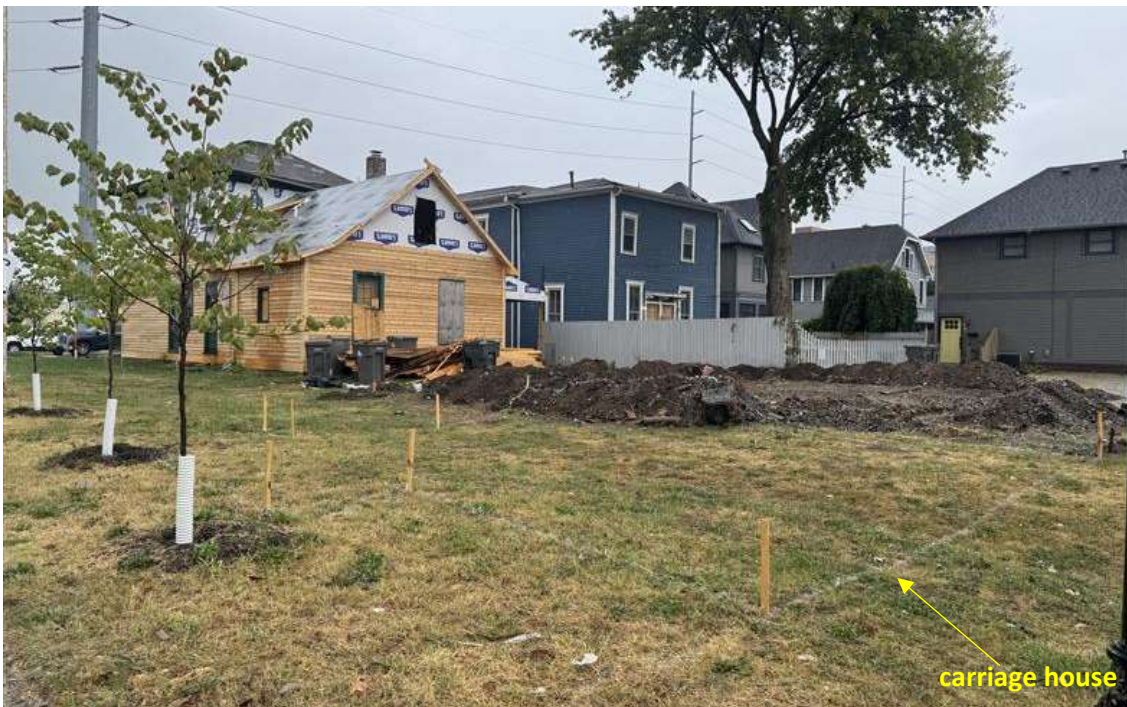
Subject property looking southeast (staking showing footprint of proposed structures)
