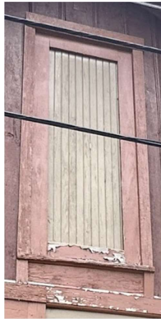
Existing hayloft opening on west/alley side
