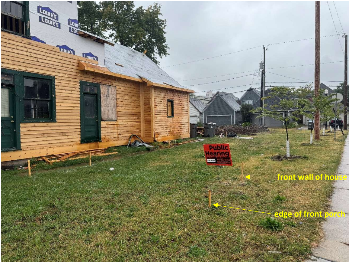
Subject property looking southwest (staking showing footprint of proposed structure)
