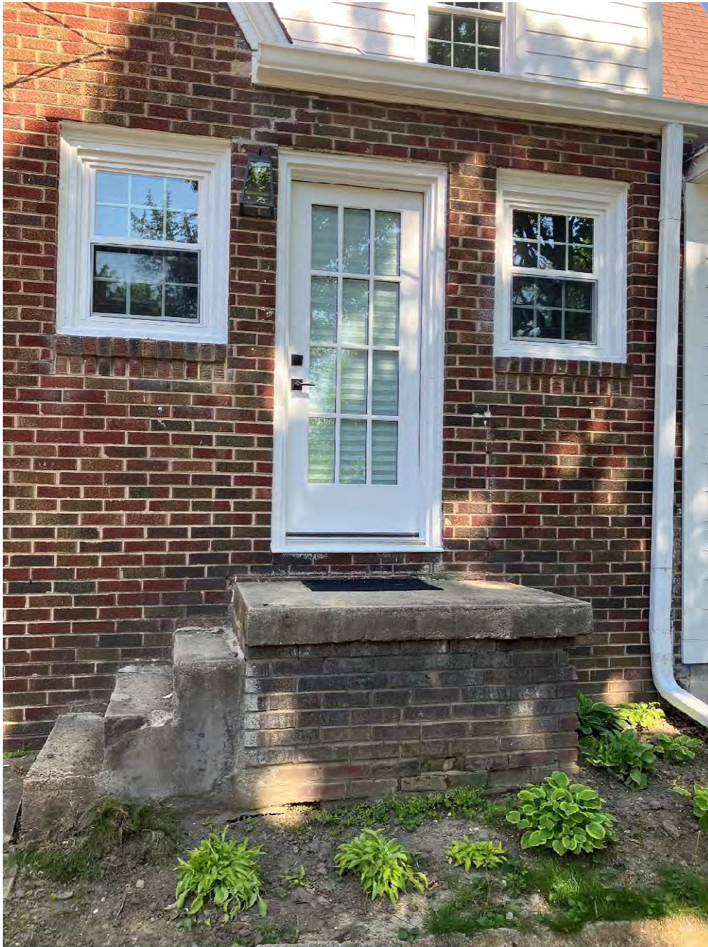
Photo 12 a: new fiberglass over wood core door - this and all exterior doors are a match of the door IHPC approved in 2024 for the house adjacent east -
