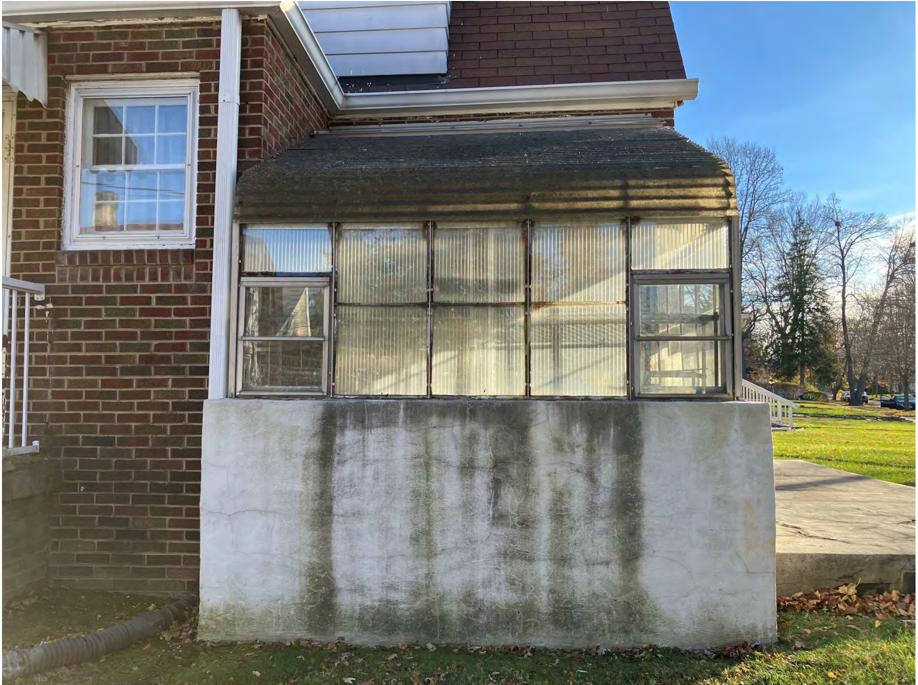
Photo 5b: Greenhouse as found - Many original windows lost & replaced with fiberglass - the stucco wall extends beyond the foundation and is built on packed earth.
