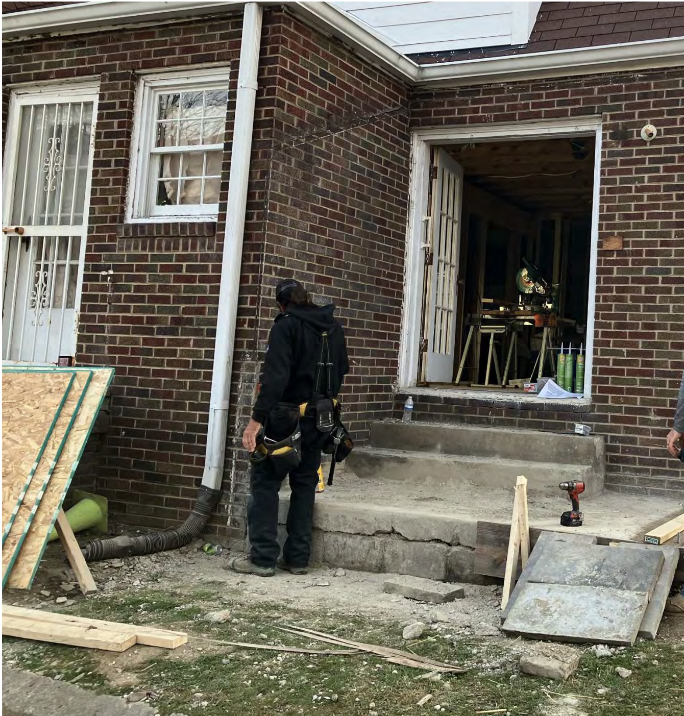
Photo 6: Greenhouse removed and original slab on concrete block on concrete footer exposed
