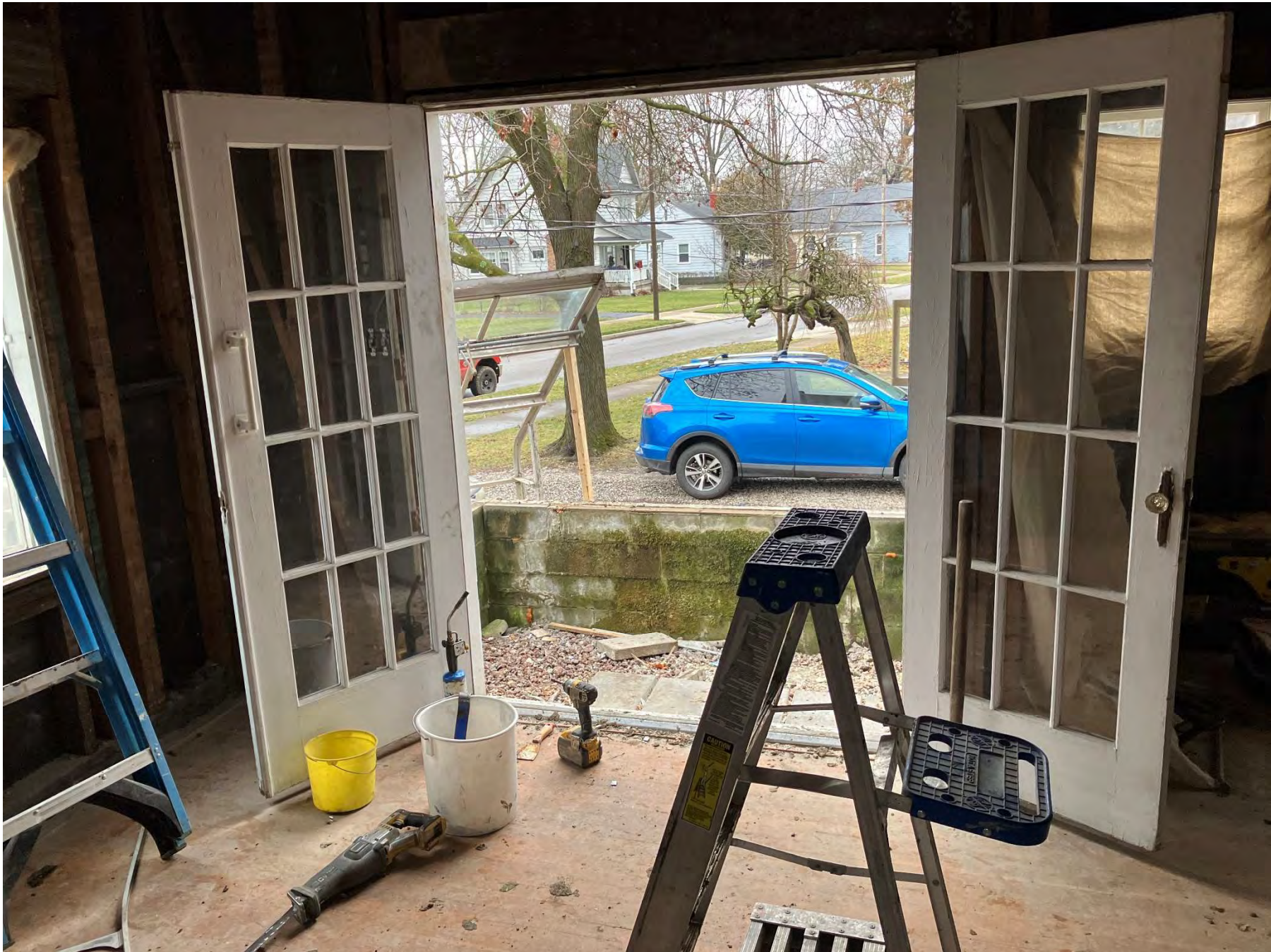
Photo 13: Greenhouse east wall after removal of aluminum & glass, showing block wall sitting outside (off) of the foundation.
