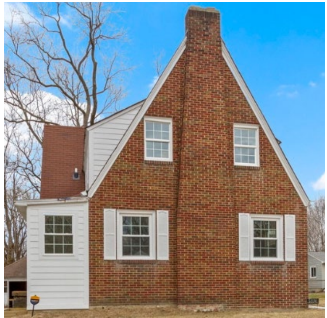
Front/South elevation (right before, left after) - showing change from 8 lite casements to 6/6 hung units
