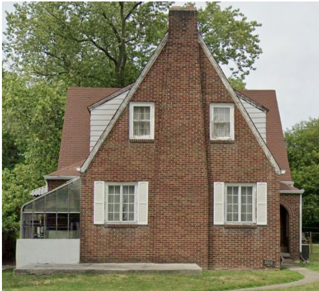
Front/South elevation (right before, left after) - showing change from 8 lite casements to 6/6 hung units
