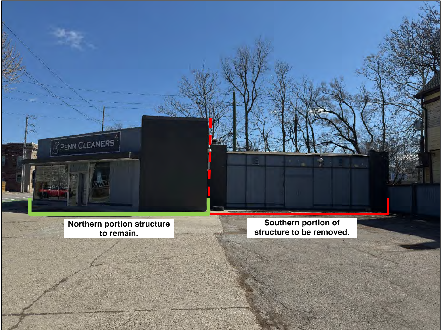
Photo 2: Western elevation of the Penn Cleaners building looking east. The red dashed line indicates the boundary of removal. The northern portion of the structure will remain. The southern portion of the structure will be demolished.
