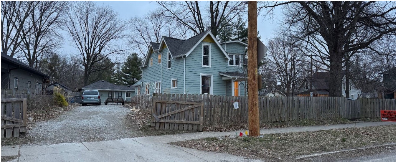
Subject property as seen from Audubon Rd with subject garage visible at the rear
