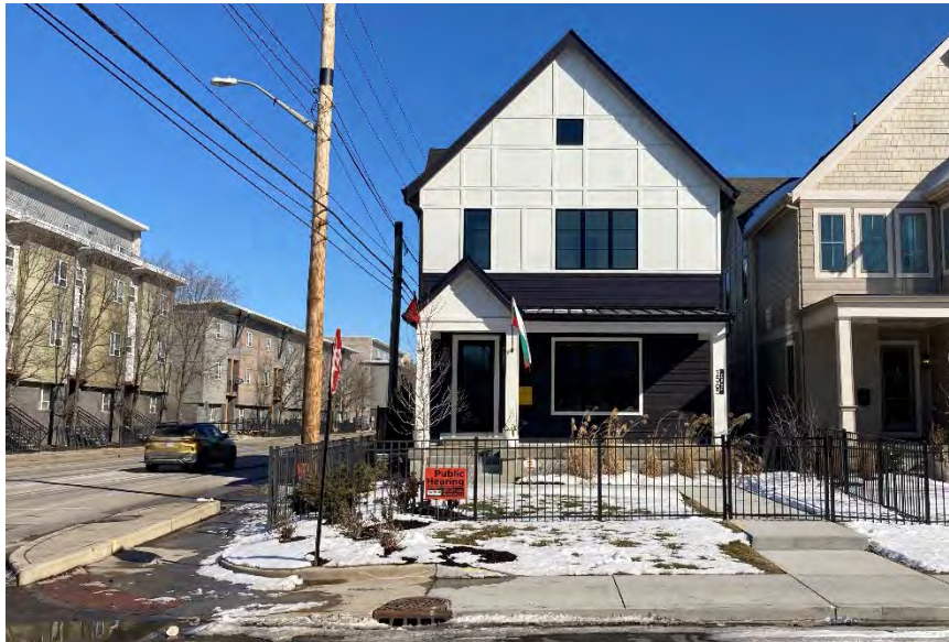
Front / west elevation – showing front yard fence and 16 th Street
