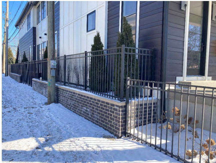
4' tall front yard fencing installed (right of image) and 24" tall landscape wall with a 4' tall fence on top of it (left of image)
