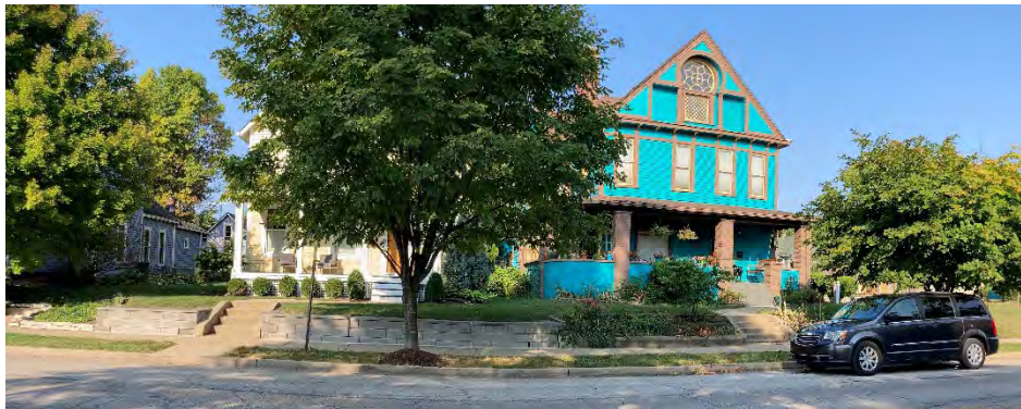
Properties to the west, across North Alabama Street
