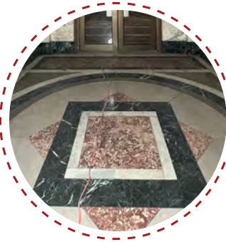
EXISTING MARBLE FLOORING
