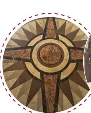
EXISTING MARBLE FLOORING
