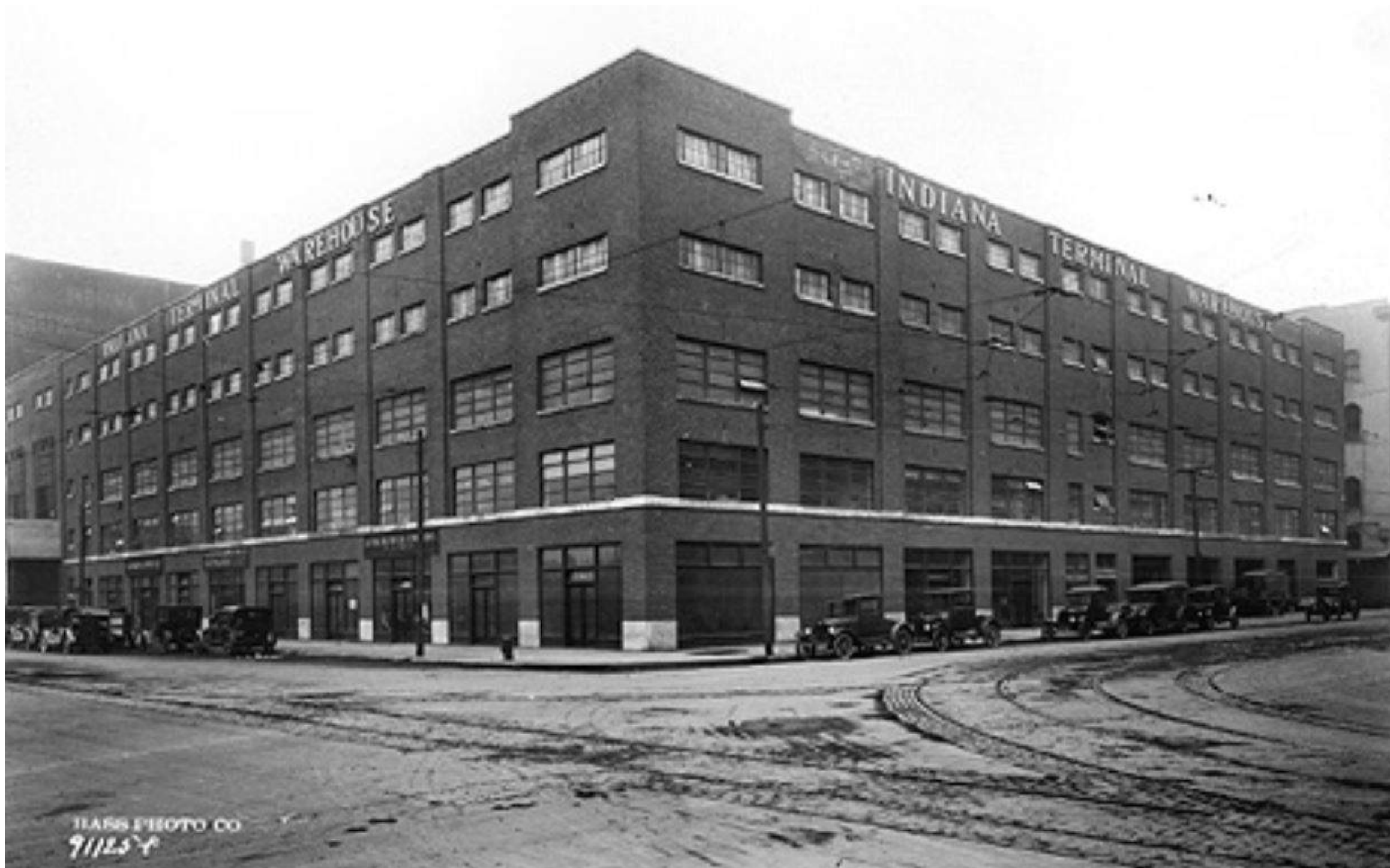
1925 HISTORIC PHOTO LOOKING SOUTHWEST
