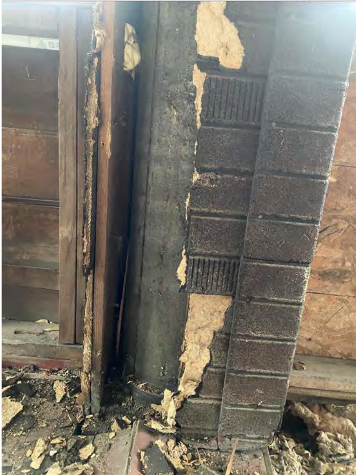
Original 2 nd Story Columns
