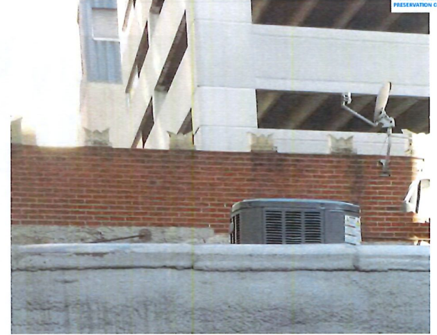
Current configuration of back-up brick in the parapet.
