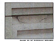
SHARD TO BE DUTCHMAN REPAIRED
