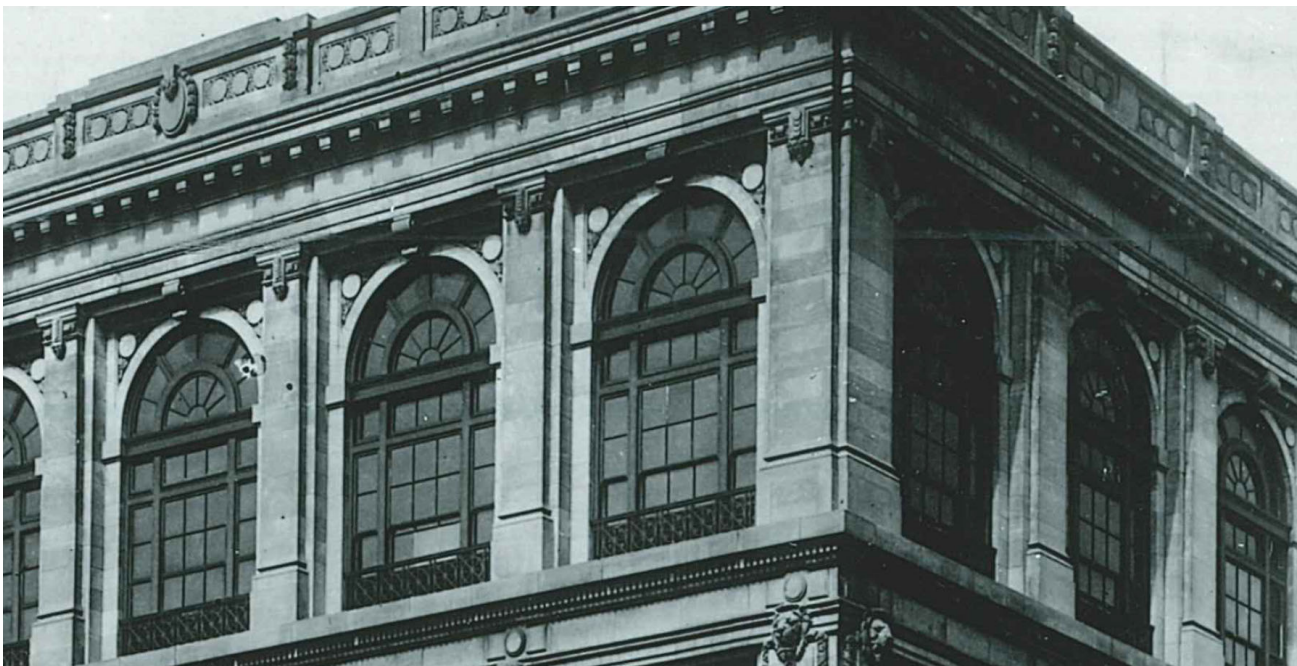
Historic window detail
