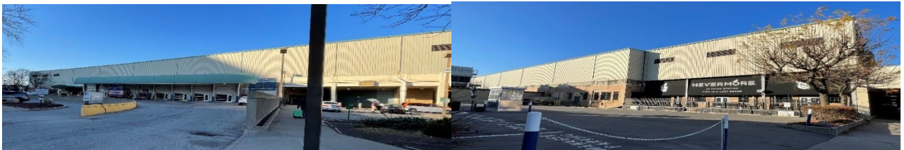
1916-1922 Concourse and Train Shed (rear/south elevations)
