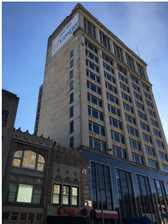
Subject properties, west façades. North façade of 1 N. Pennsylvania visible.
