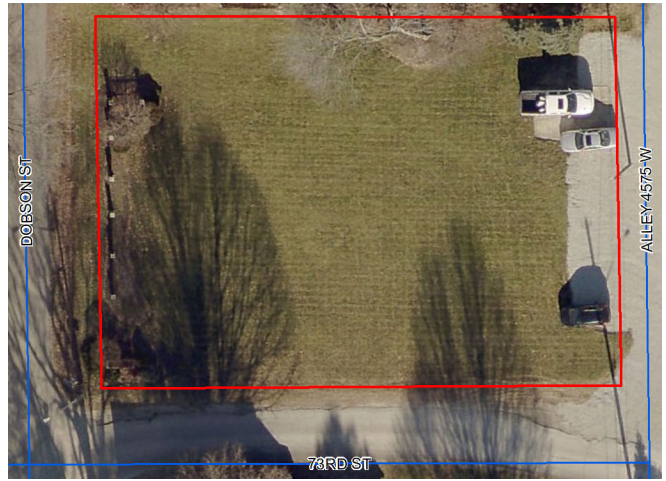
Fall 2021 – gravel has been installed
