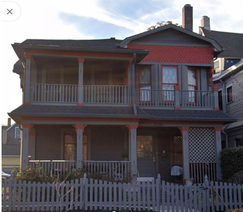
2022 Google Street View image of front (east) elevation
