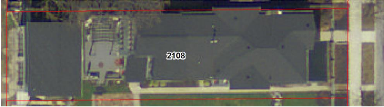
2015 aerial photo – after construction of shed-roof, enclosed porch, approved in 2014.
