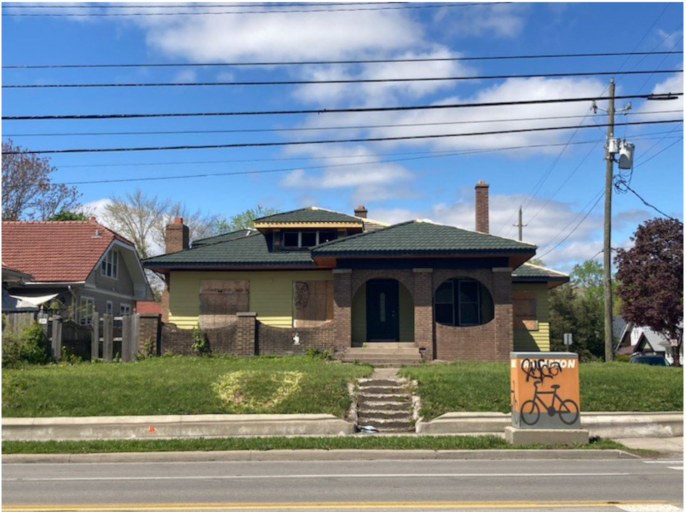
April 24 th photo of metal roof installed
