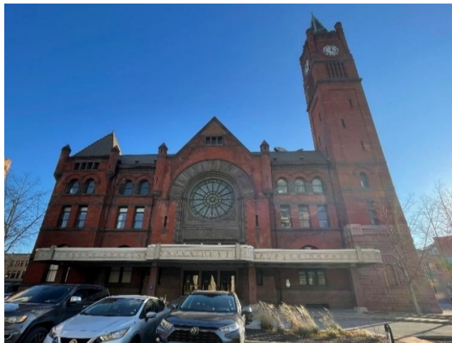
1888 Union Railway Station (north elevation)
