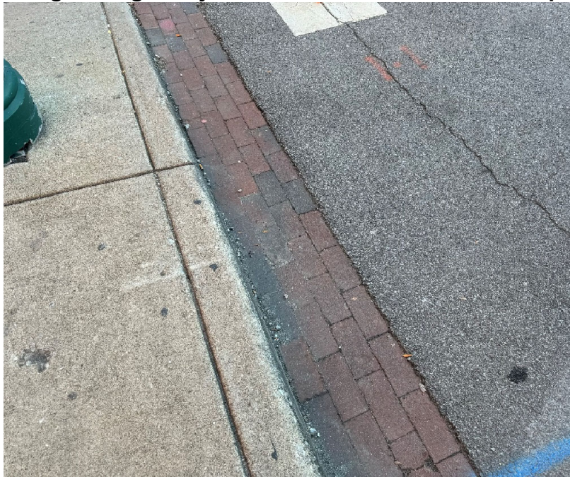
Existing brick gutter just north of Illinois Street underpass
