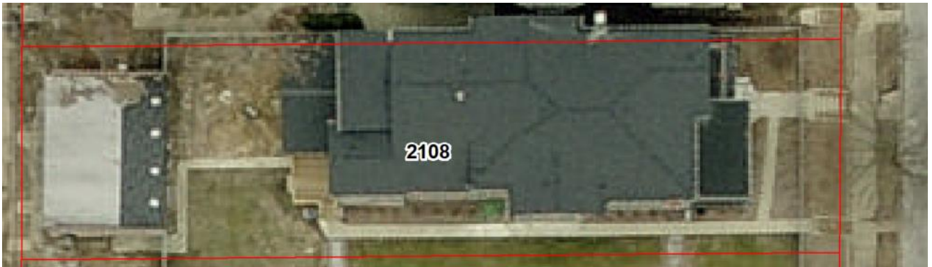
2008 aerial photo – after construction of first-floor, 1-story, addition approved in 2007.
