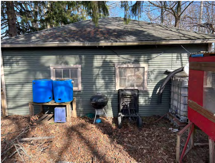
Outside view of South Wall:
