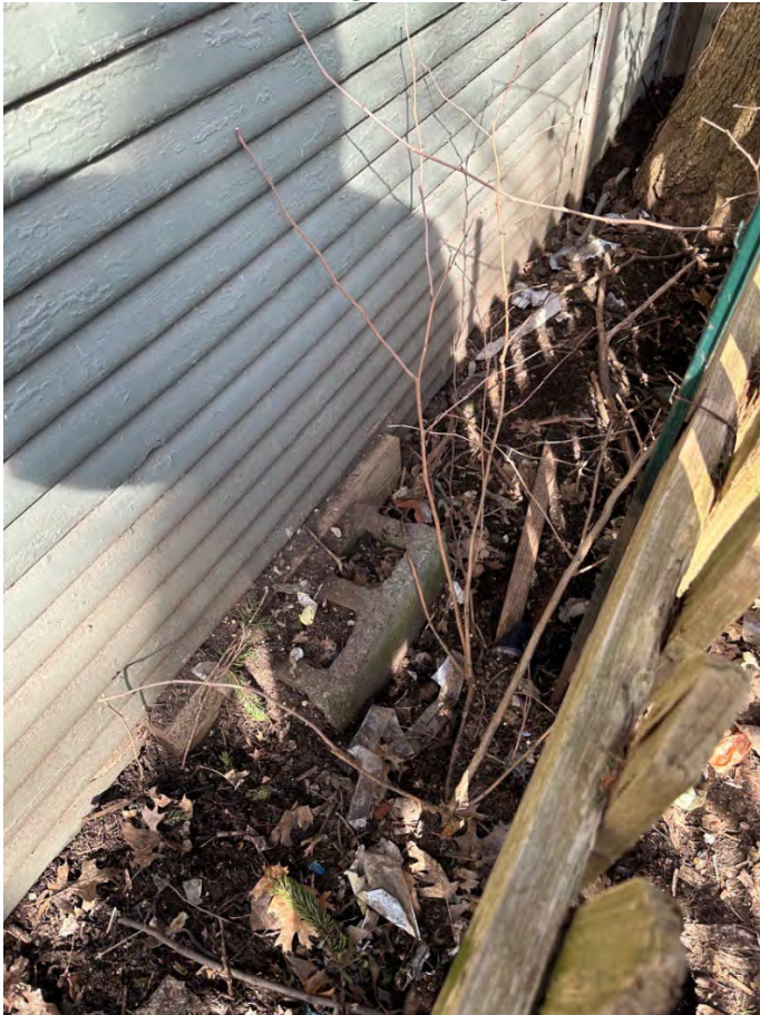
Outside of East wall, dirt against siding and holes in wall.
