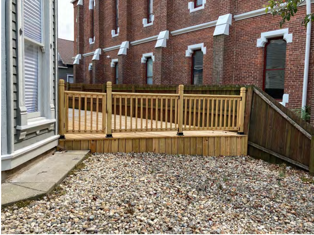
July 2021. Deck before fence installation.
