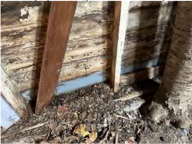
East Wall condition displaying termite damage to frame, rotted clapboards, baseboard termite damage/rotted. Unsteady replacement pieces and additional pieces to shore up damage.
