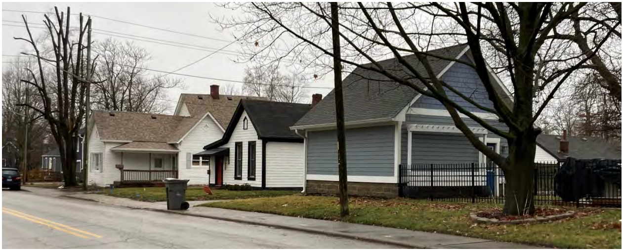
Garage with context to the south
