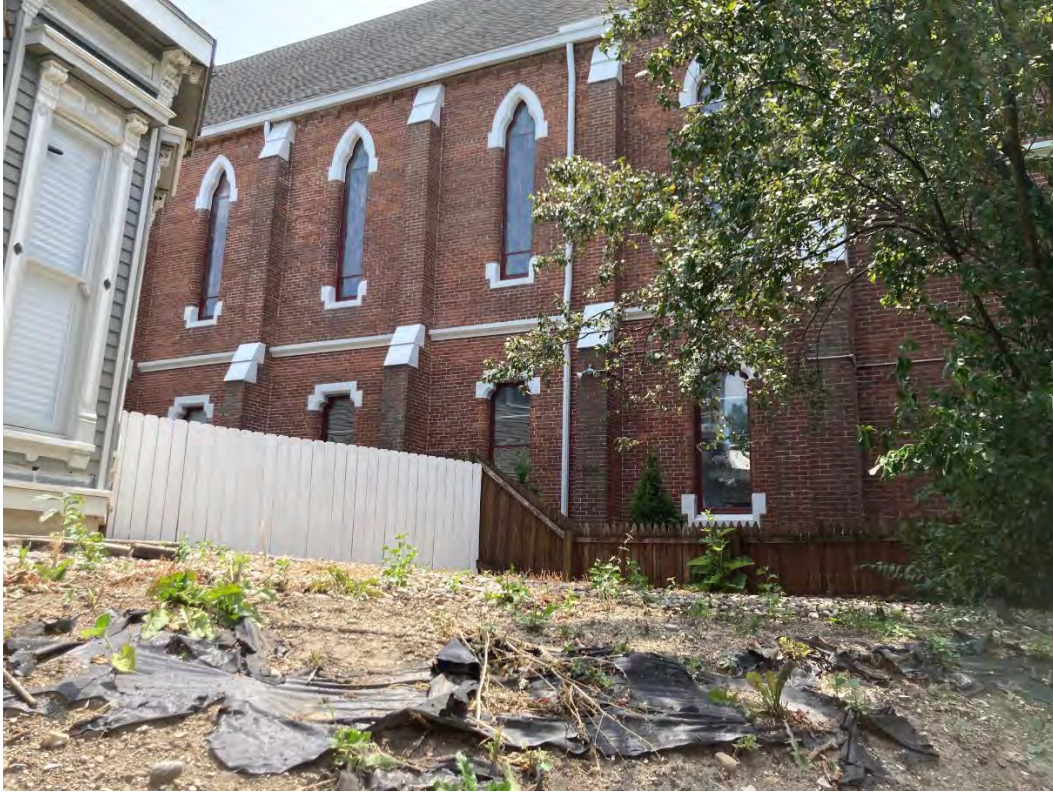
June 2023. Deck located behind white fence.
