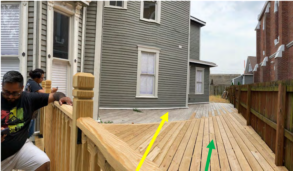
July 2021. Showing existing deck and deck extension.
