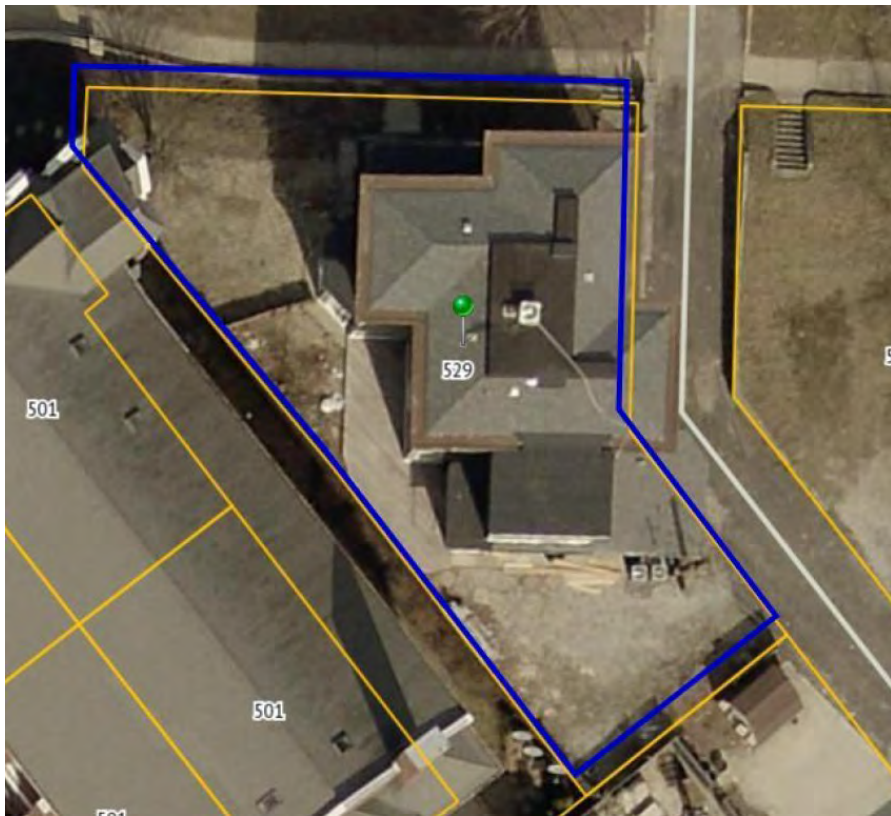
March-April 2021 aerial photo before deck extension
