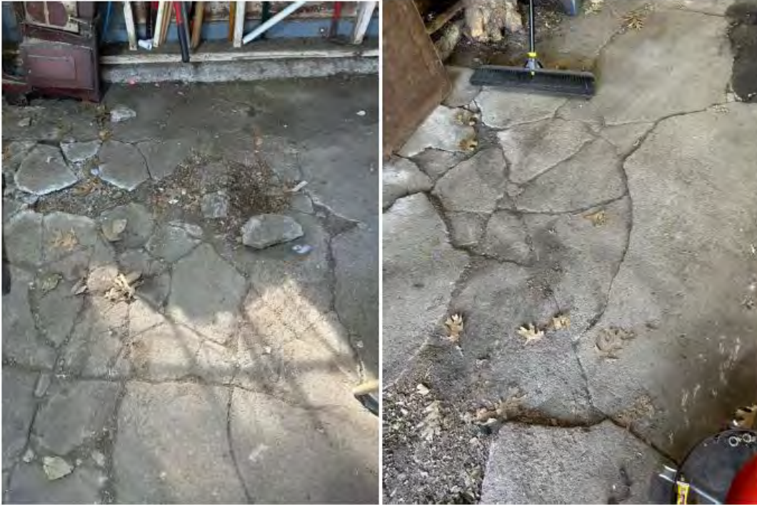
Interior Slab Conditions:
