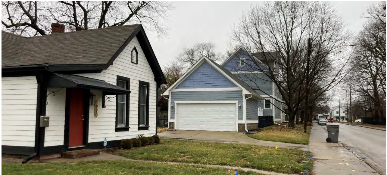
Historic neighboring cottage in foreground, with subject garage beyond
