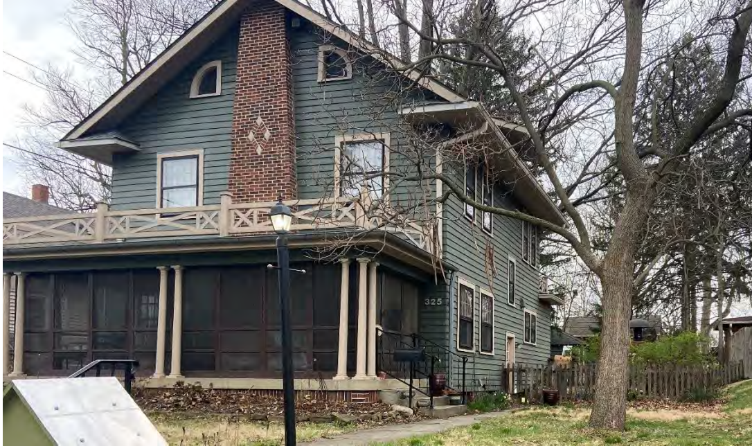
Front (west) elevation of historic house at subject property
