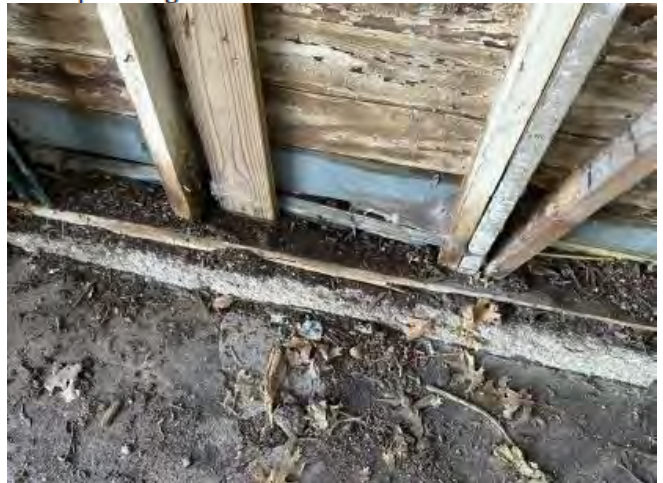
East Wall condition displaying termite damage to frame, rotted clapboards, baseboard termite damage/rotted. Unsteady replacement pieces and additional pieces to shore up damage.
