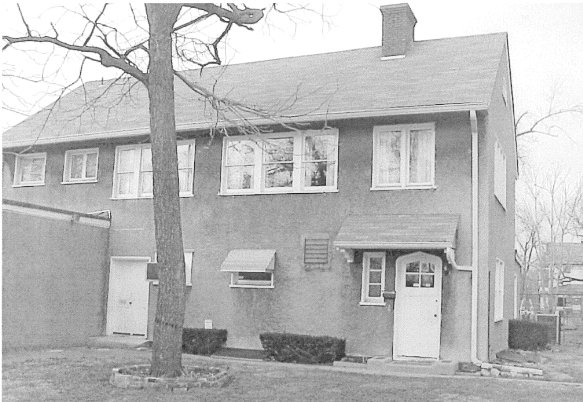
South façade before IHPC approved addition, 2002
