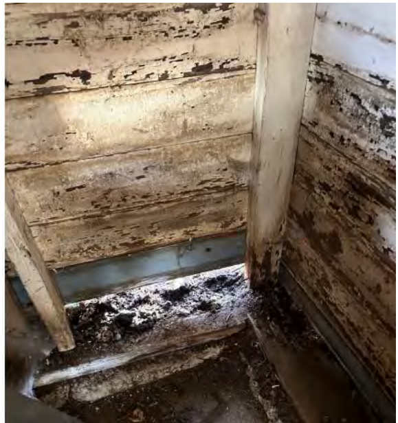
South wall crumbling foundation and remains of former support. Termite damage and rot present.
