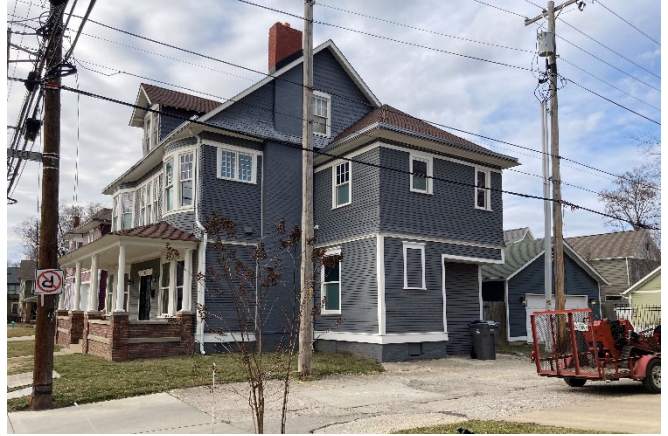
Existing east elevation – view from street
