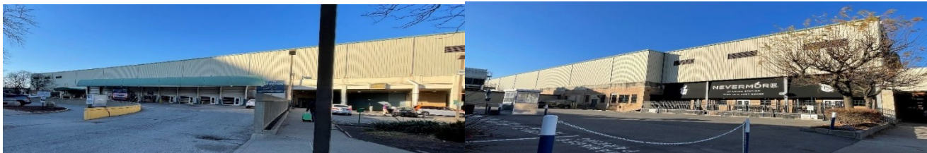
1916-1922 Concourse and Train Shed (rear/south elevations)
