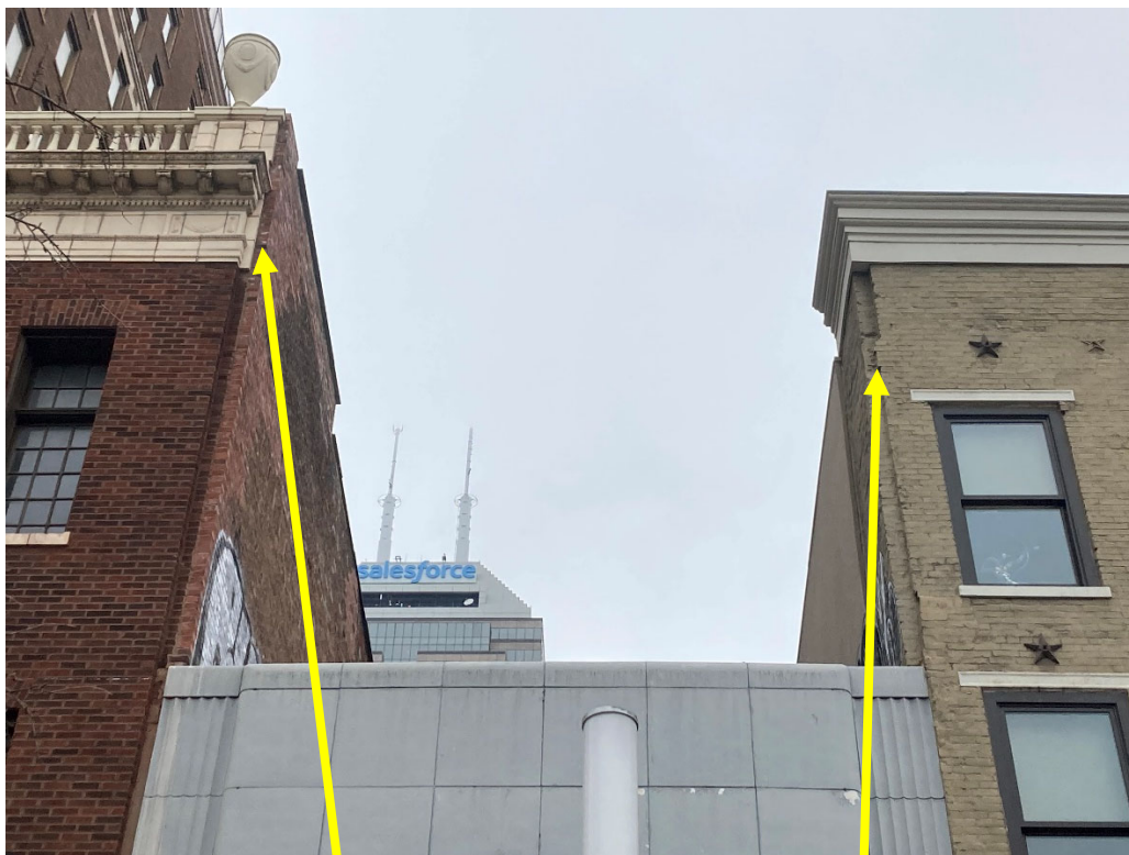
Evidence of original building height and cornice
