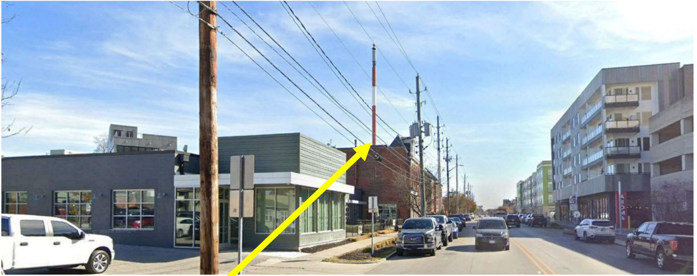
Existing pole looking southeast from Virginia Ave.
