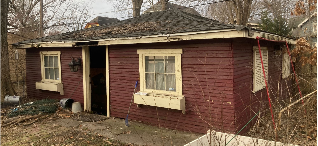
North and east façades
