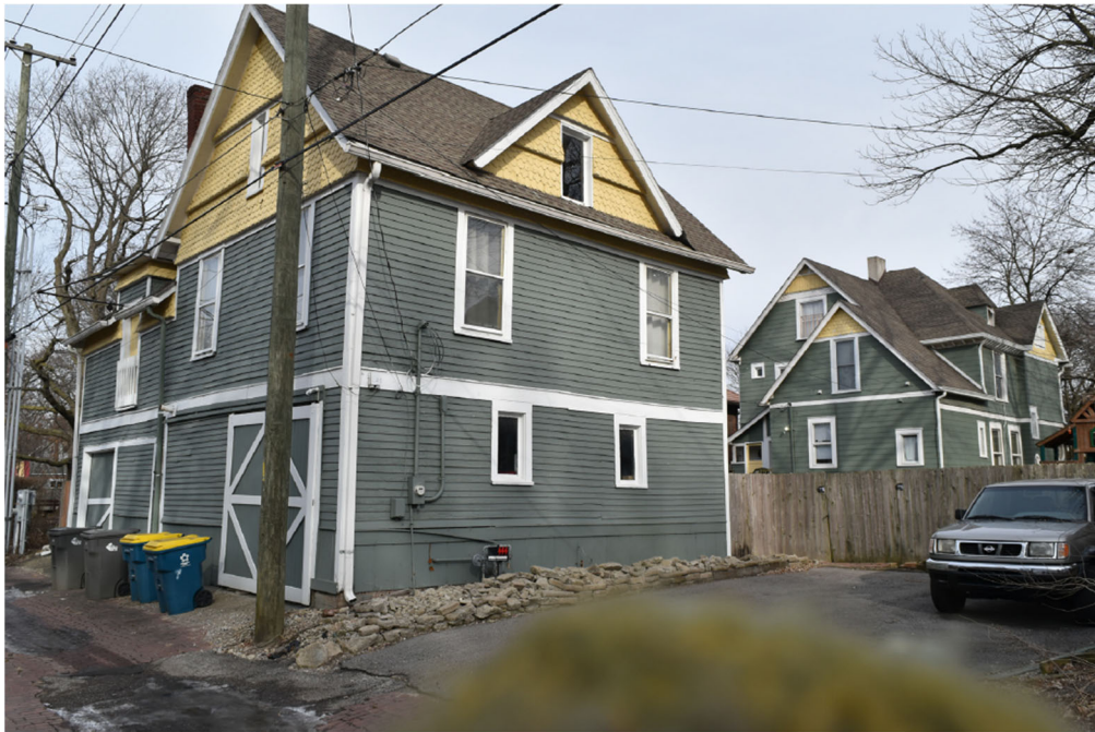
4 Existing carriage house // N of subject property
