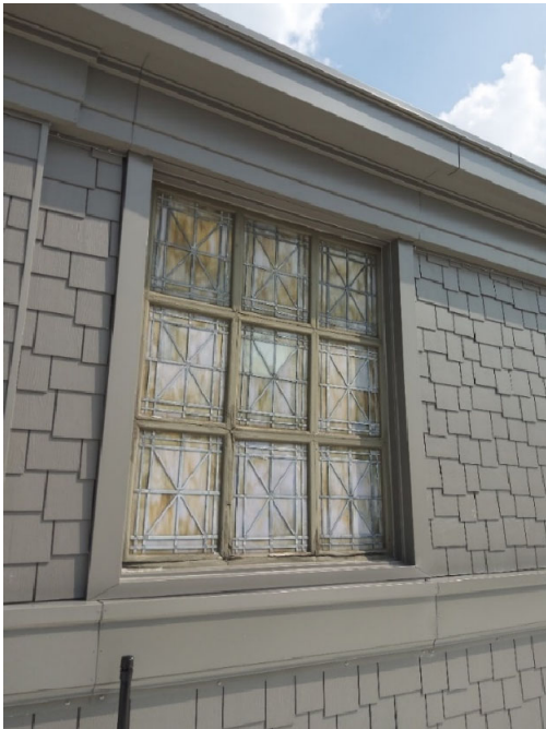
View of siding and cornice installed
