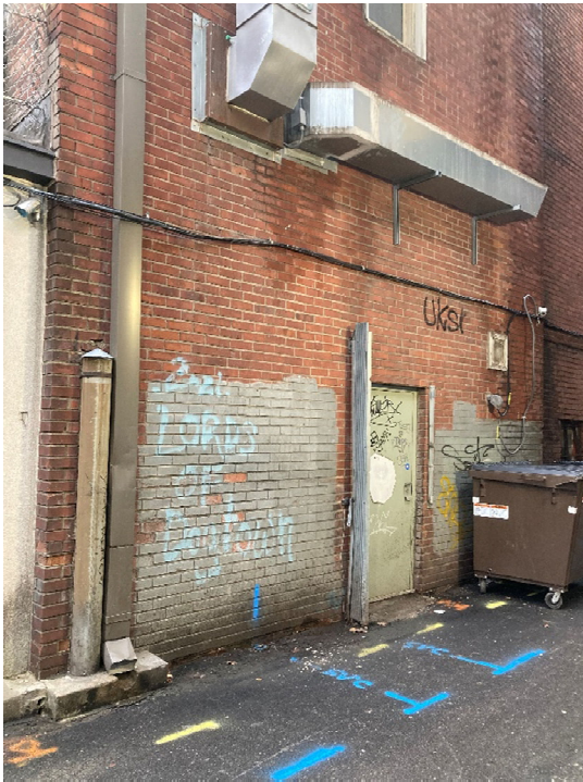
First floor of rear (north) elevation
