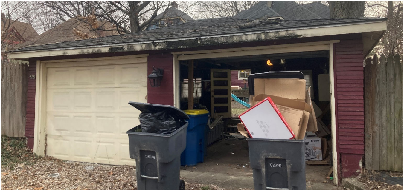
West (alley) façade
