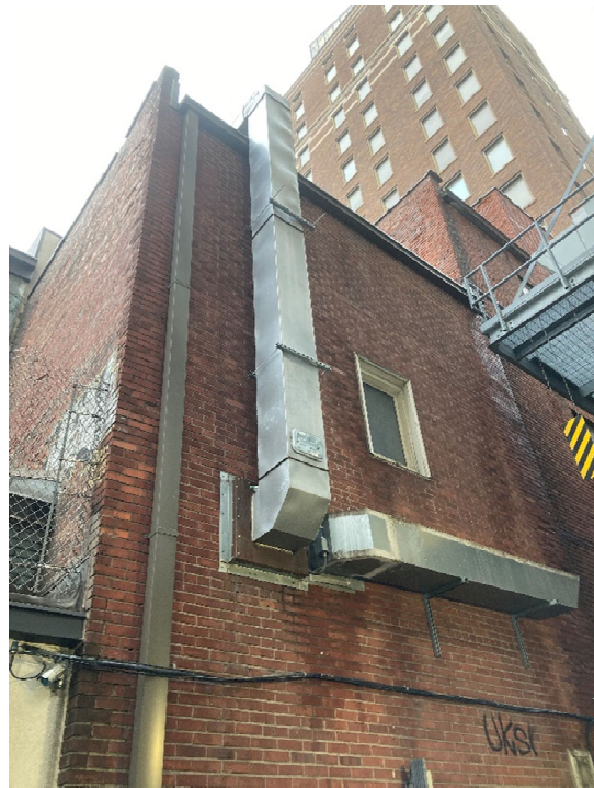
Second floor of rear (north) elevation
