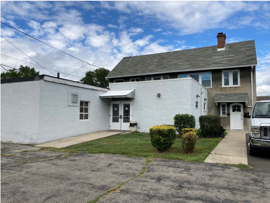
South façade with coated concrete block additions (1940s/50s, left and 2003, right)
