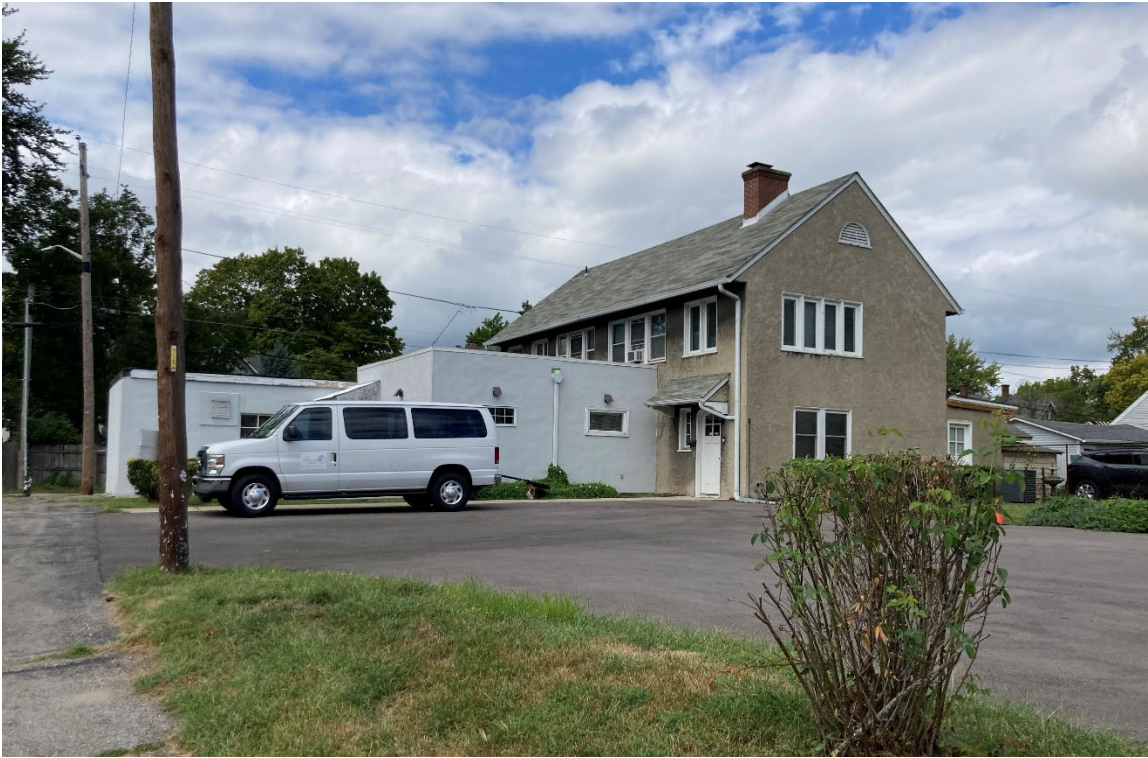
Subject property, with south and east facades visible
