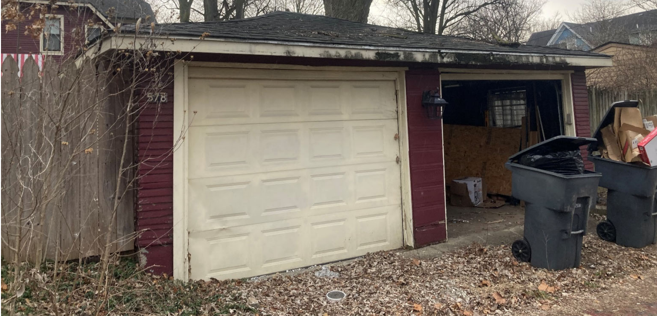
West (alley) façade
