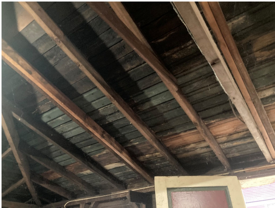
Old car siding is being used as roof decking.
