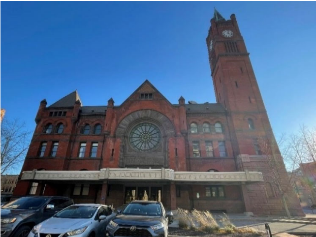
1888 Union Railway Station (north elevation)
