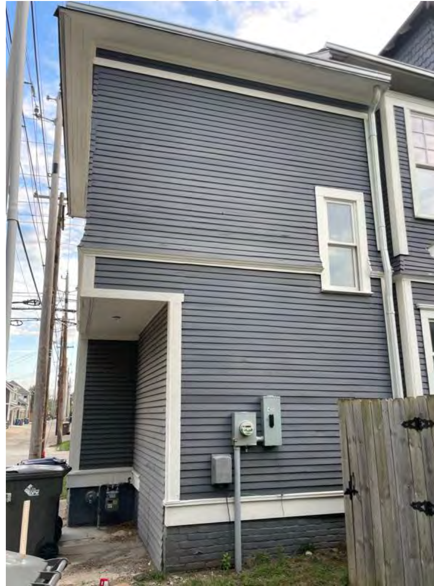
11 North east elevation at renovation area facing south
