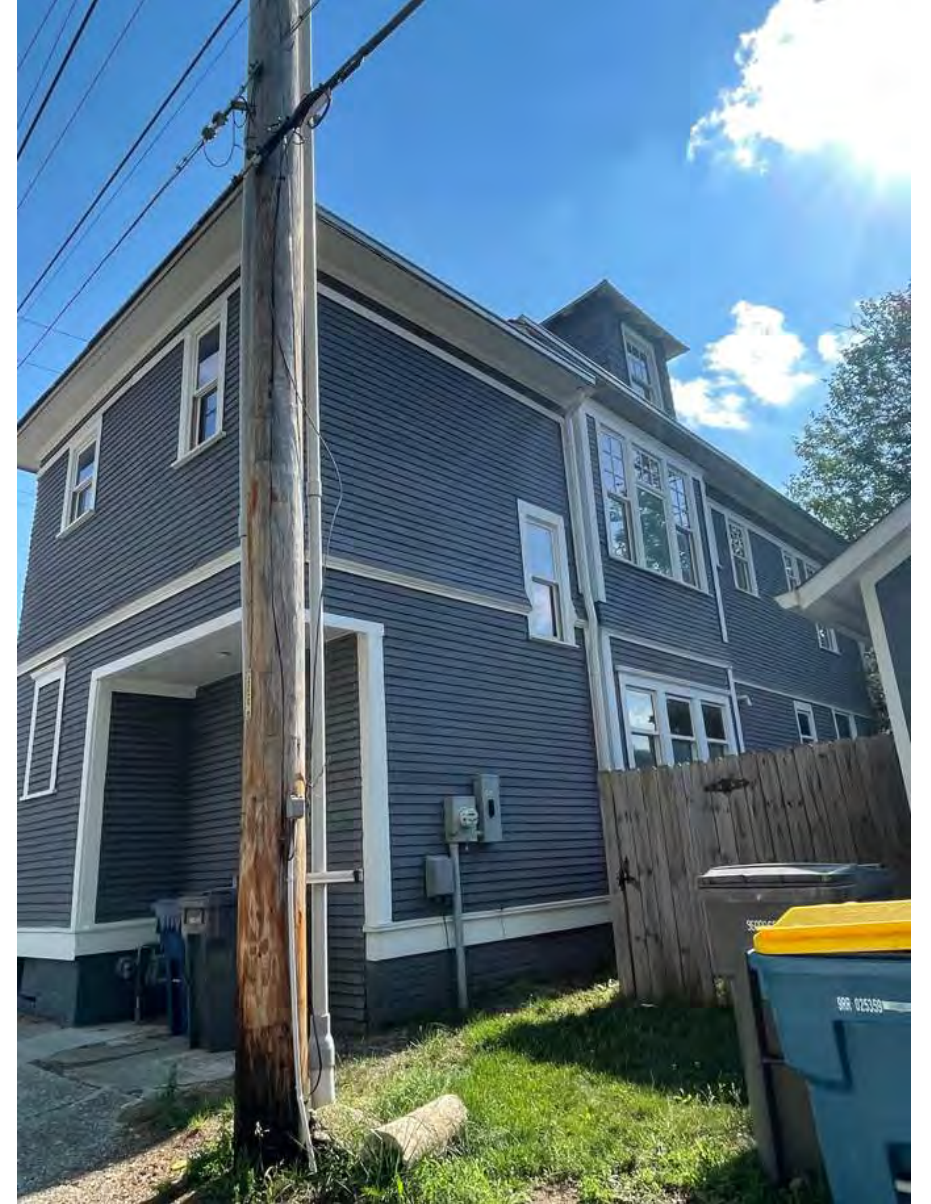
12 North east corner facing south west
