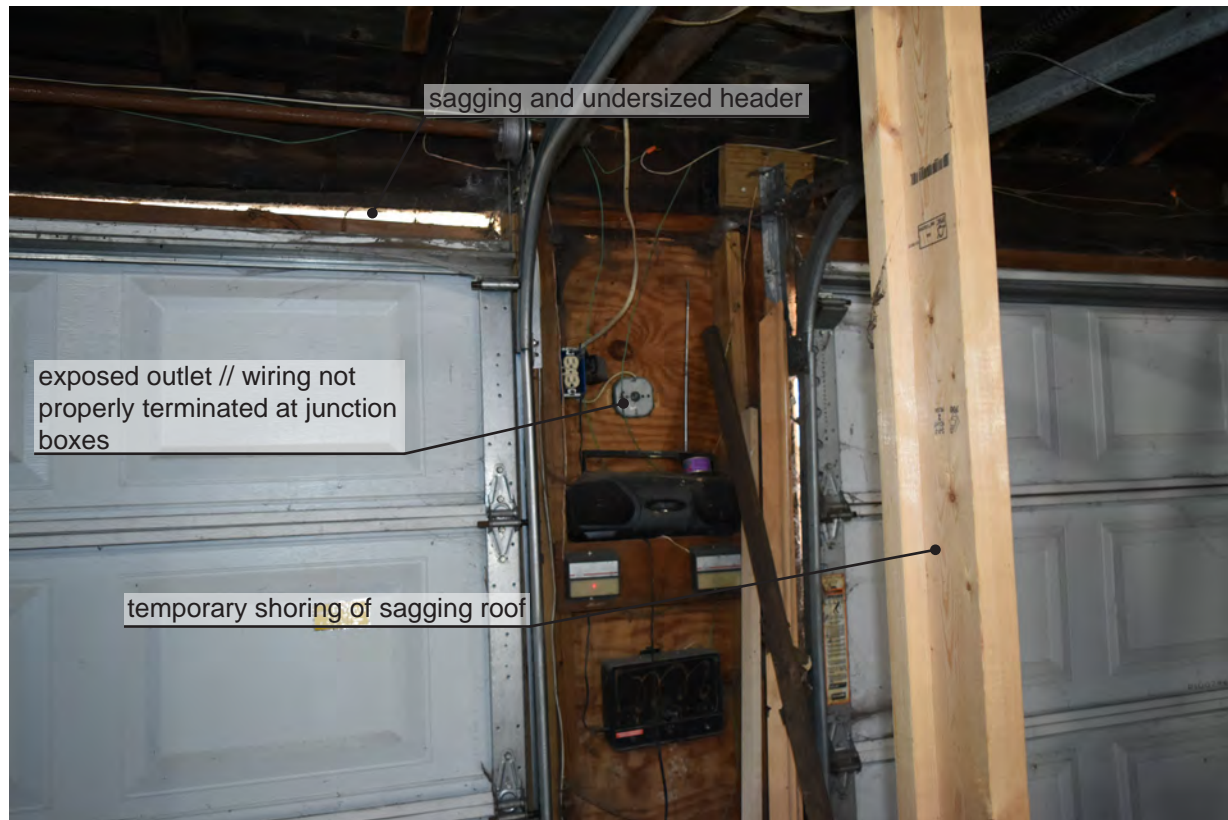
3 7 Garage interior // W wall of garage
