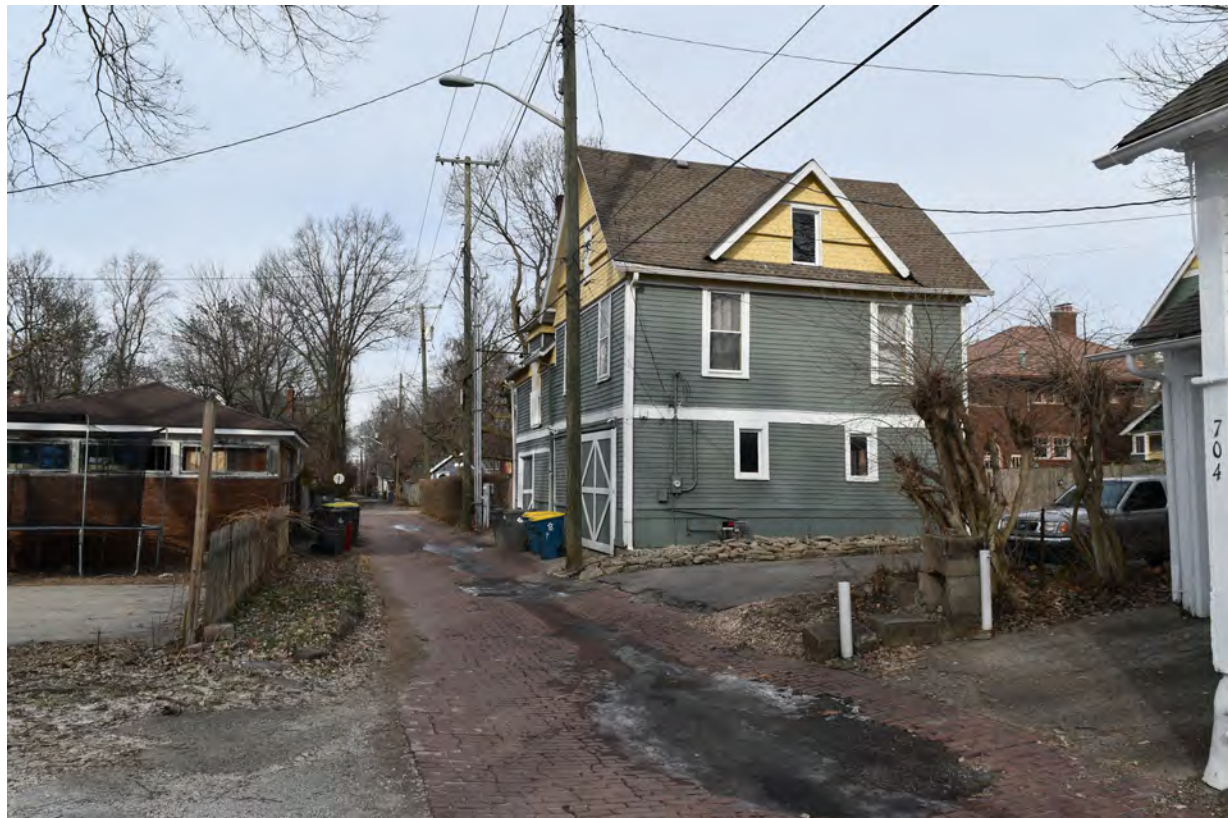
3 Existing carriage house // N of subject property 3
