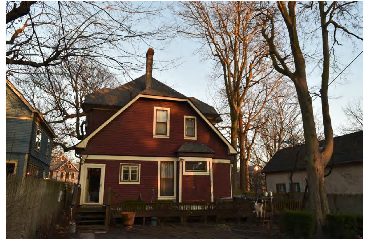
2 West facade of main house 17
