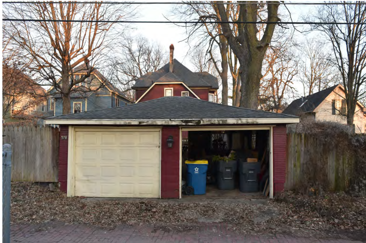
3 West facade of garage 17
