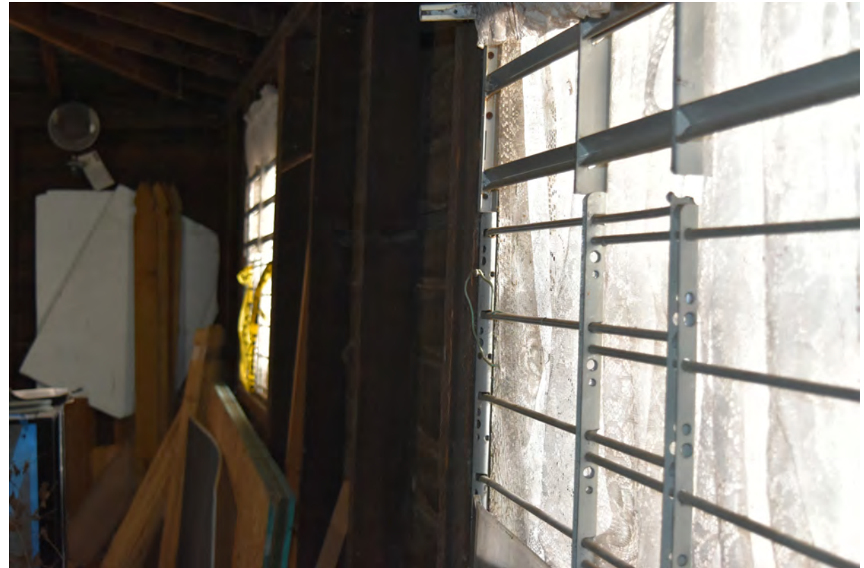
4 6 Garage interior // window facing main house
