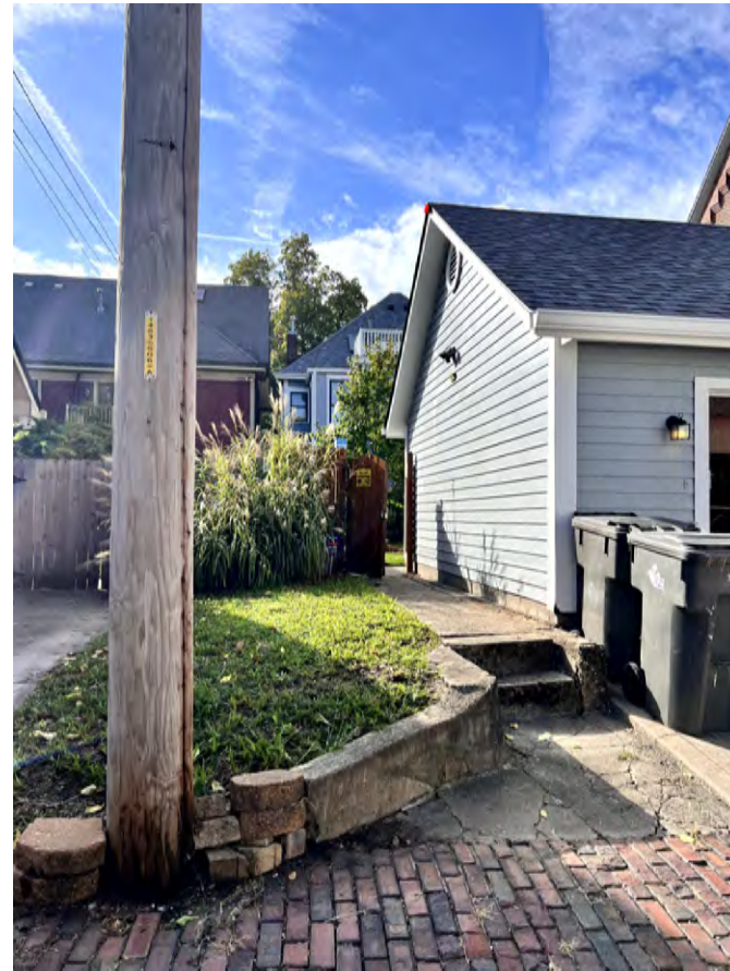
③ Existing Conditions: East Perspective of Existing Garage Scale: N/A
