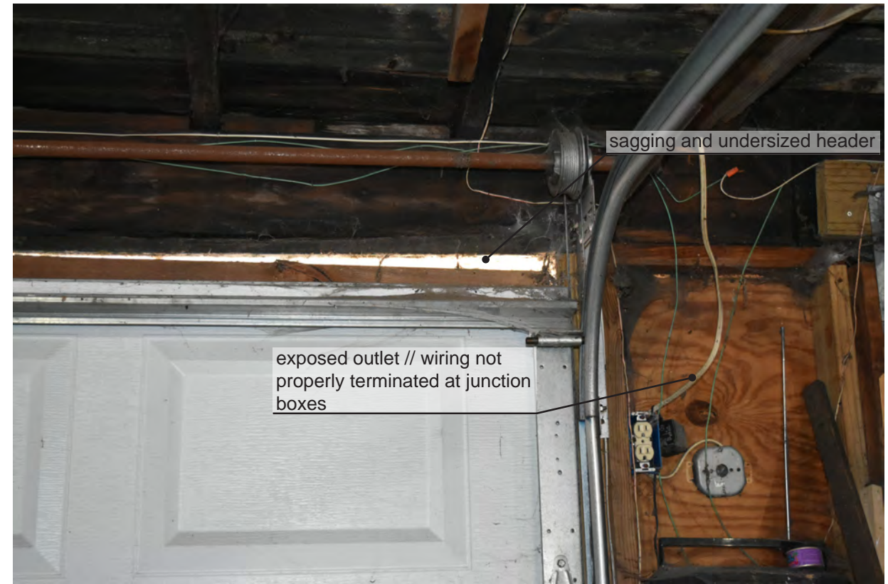
2 7 Garage interior // W wall of garage
