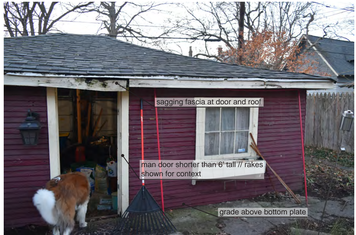
4 18 East facade of garage
