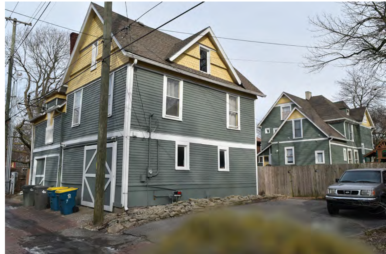
4 Existing carriage house // N of subject property 3
