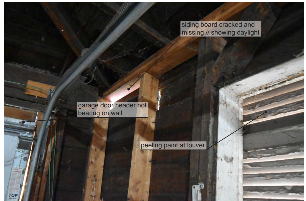
4 7 Garage interior // N wall of garage
