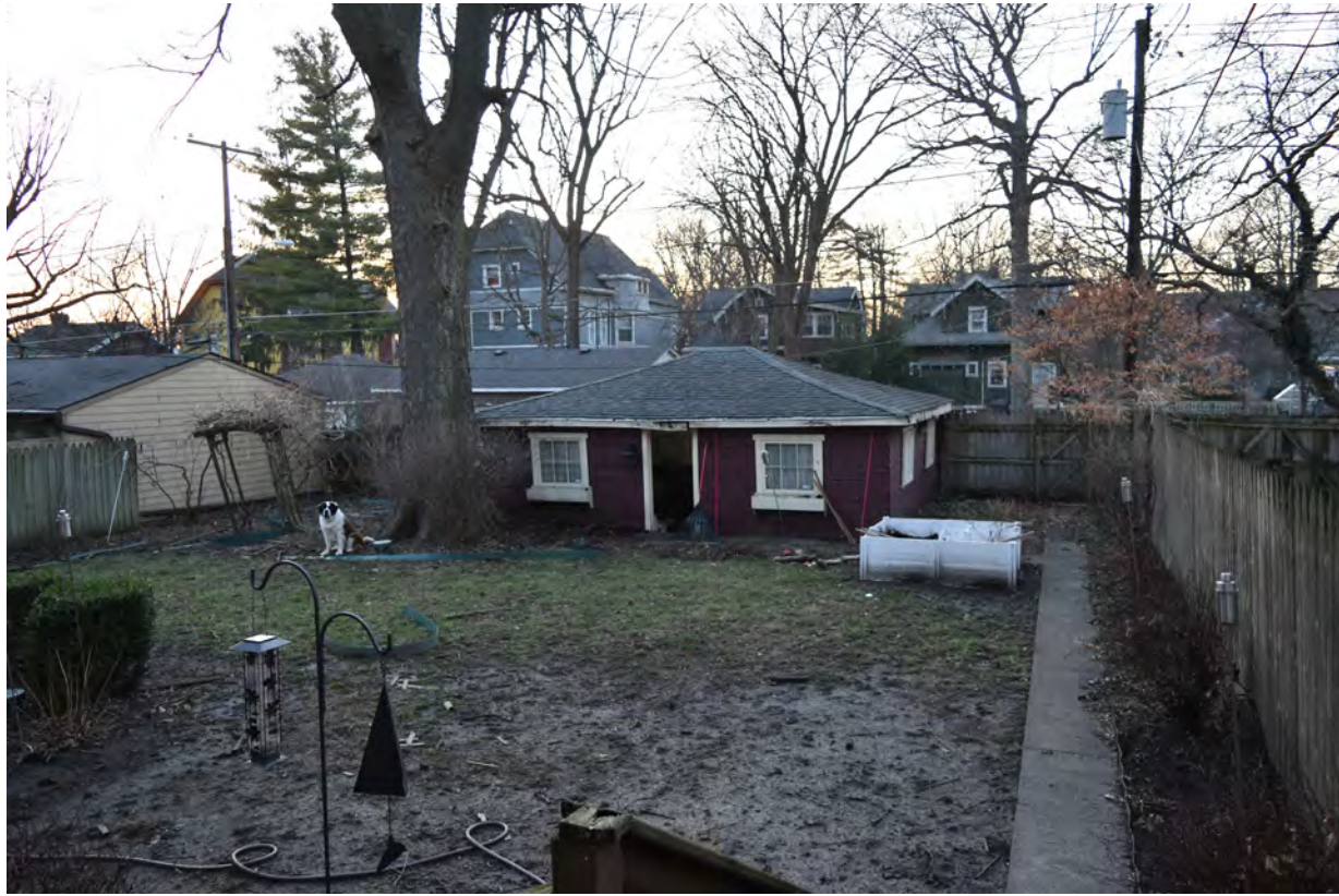
1 20 View of east facade of garage
