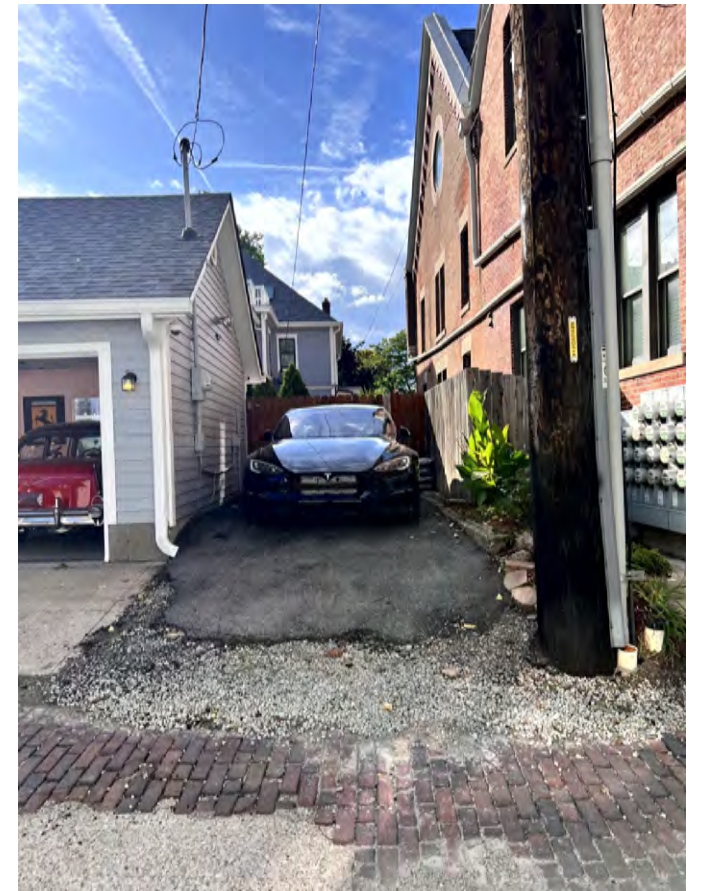
④ Existing Conditions: East Elevation of Existing Garage and House Scale: N/A
