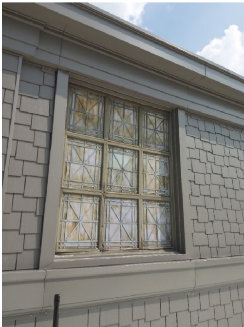
View of siding and cornice installed
