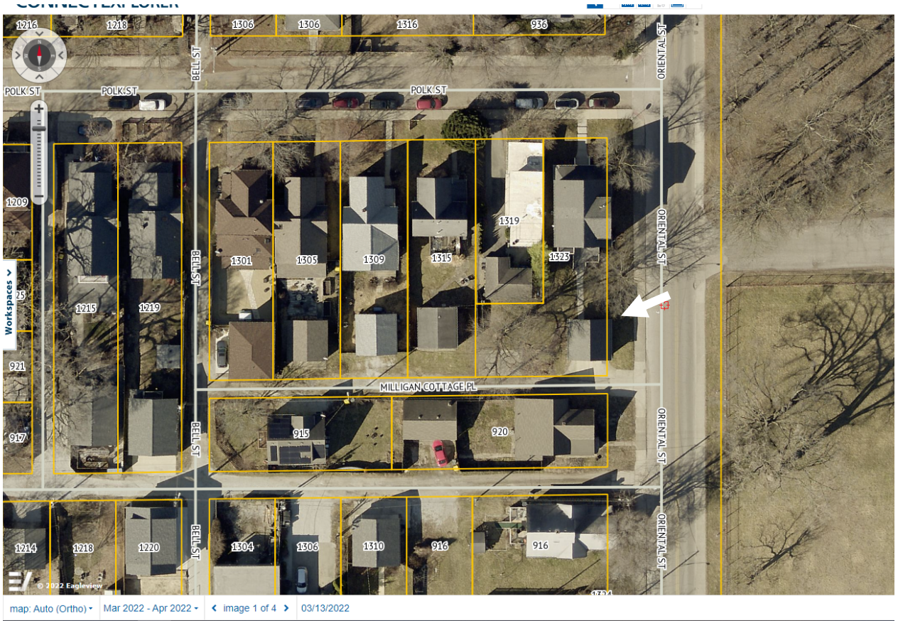
Aerial view, subject garage indicated by arrow
