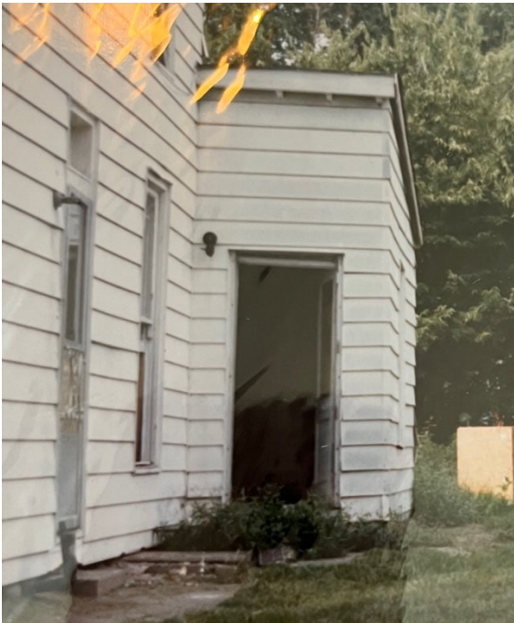
South elevation of addition
