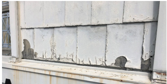
Shingles that were replaced
