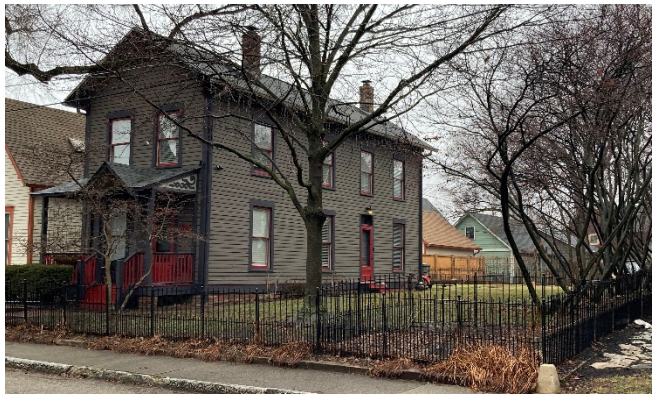
Subject property – view of south and east elevations, showing visibility of location where addition and garage would be constructed.
