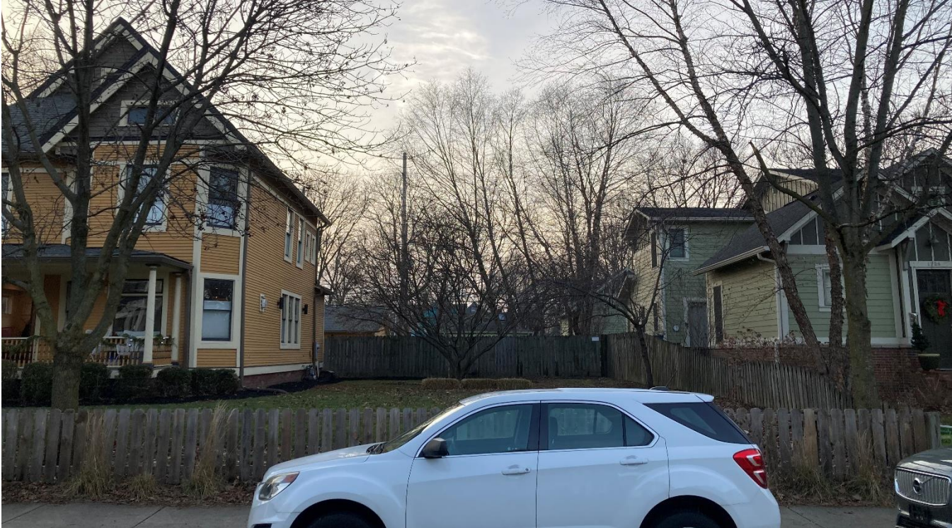
Looking west at subject site
