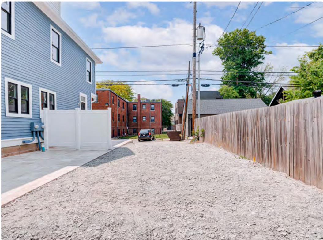
2023 listing photo of rear yard looking west, prior to installation of sod.
