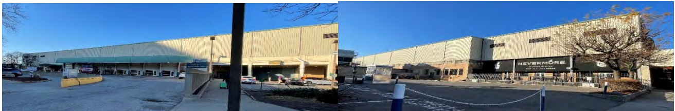
1916-1922 Concourse and Train Shed (rear/south elevations)
