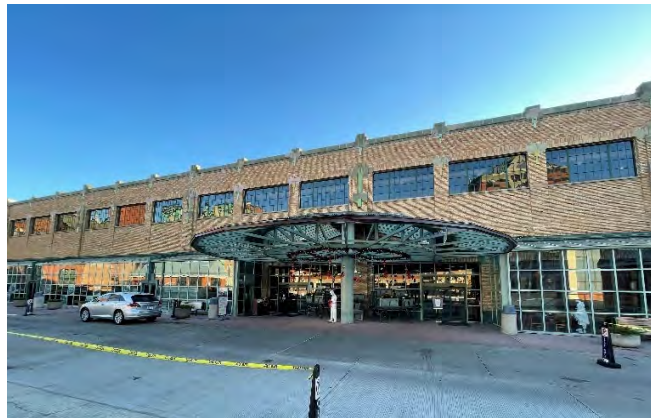
1916-1922 Concourse and Train Shed (north elevation, between Illinois and Capitol)
