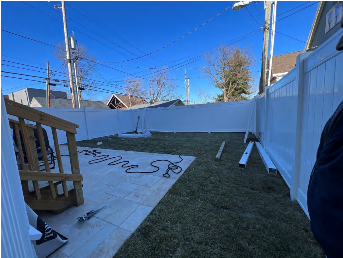
Looking north at finished backyard space on 320 side of duplex.
