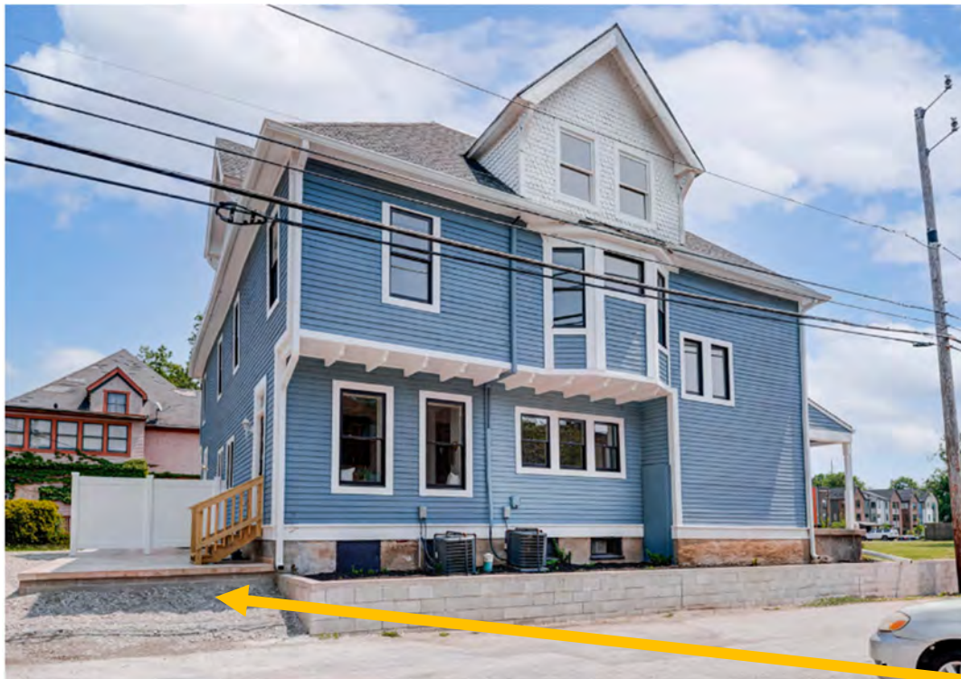
2023 listing photo of rear (north) and west elevations. Retaining wall extension to be here.
