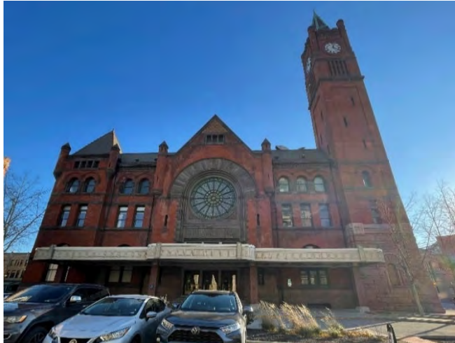
1888 Union Railway Station (north elevation)
