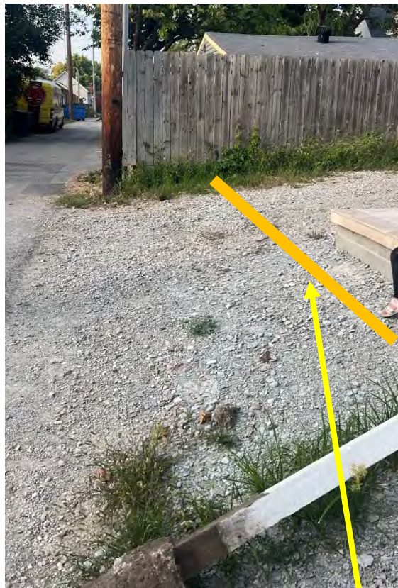
Looking north. Retaining wall extension to be here (approximately).
