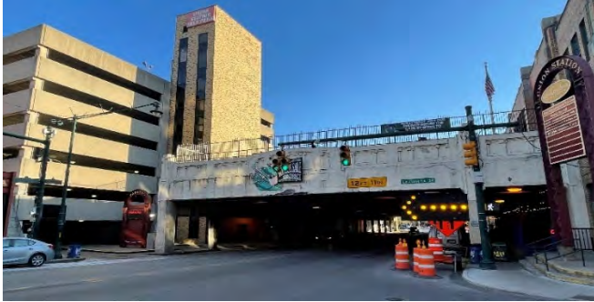
Meridian Street Bridge (left north elevation, right south elevation)
