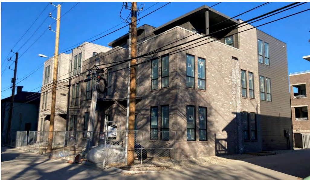
Duplexes under construction, subject lot at far end of construction site
