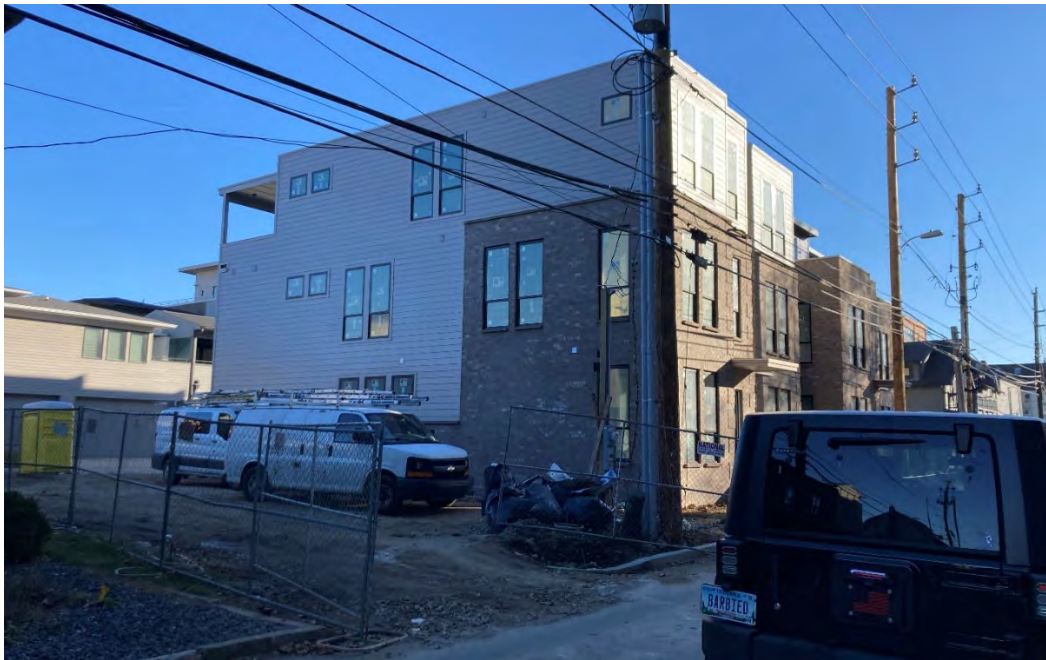
Duplexes under construction, with subject lot visible in the foreground
