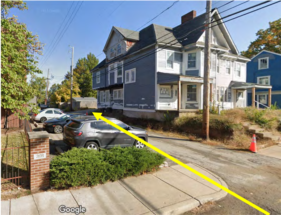
2022 Google Street View during renovation. Location of wall extension here.
