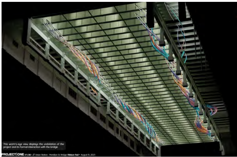
Overall view of installation with color variation one
