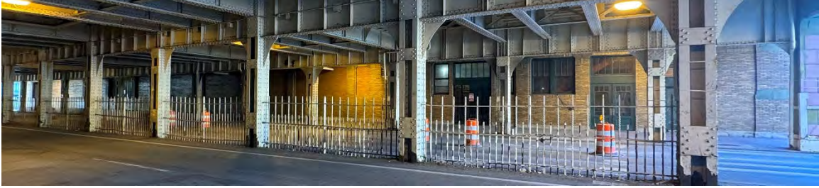
West side of Illinois Street underpass
