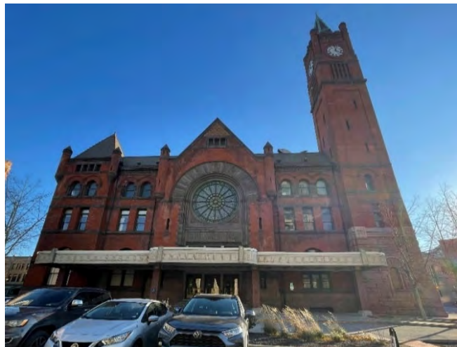
1888 Union Railway Station (north elevation)
