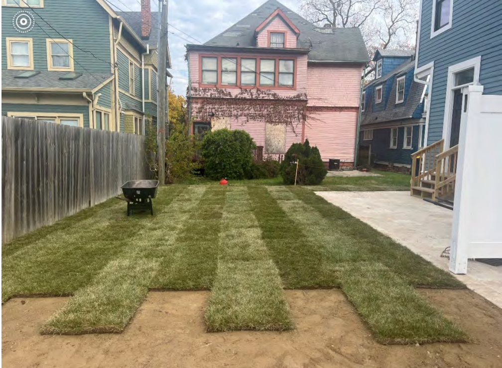
Rear yard looking east during sod installation.
