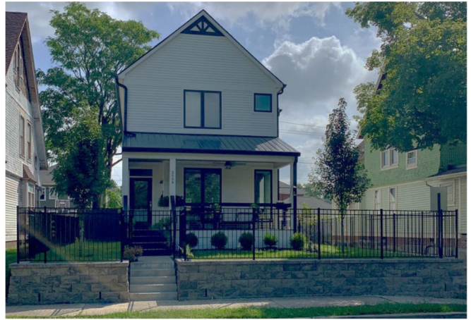
2009 N. Pennsylvania – retaining wall & fence installed without approval
