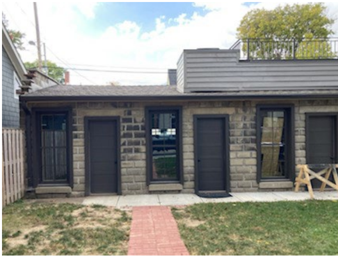
East side of concrete block garage addition
