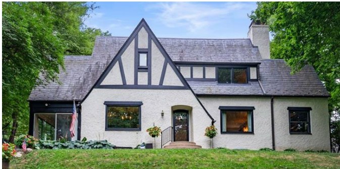
View of front/north elevation of house
