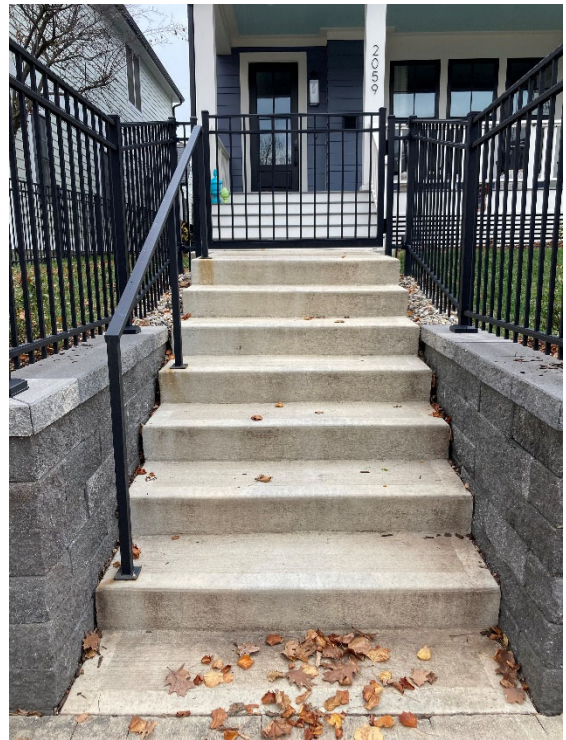
Existing stairs and fencing
