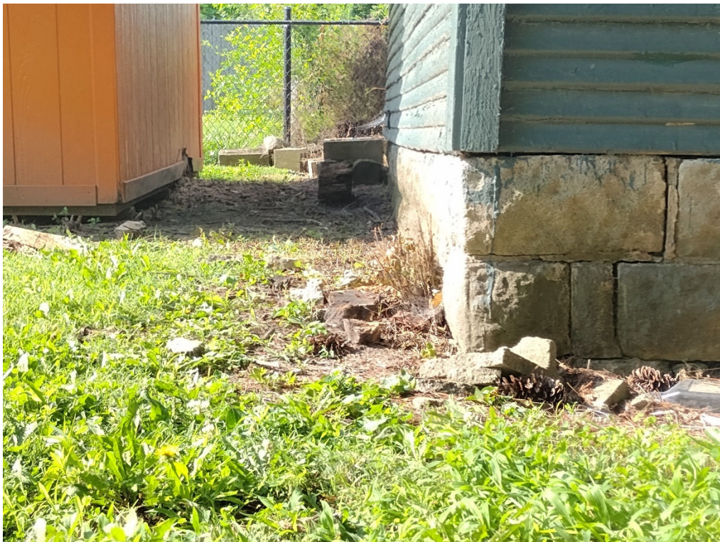
Examples of out of plumb foundation and exterior wall
