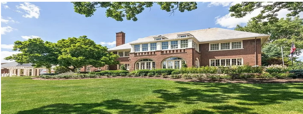
Photograph of 3148 N Pennsylvania Street
