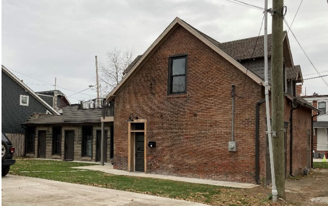
Subject property – east elevation
