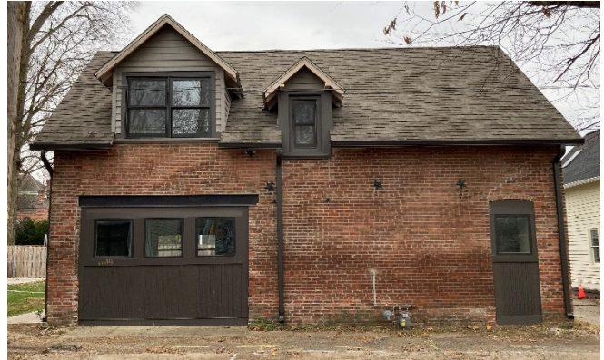
Subject property – north elevation
