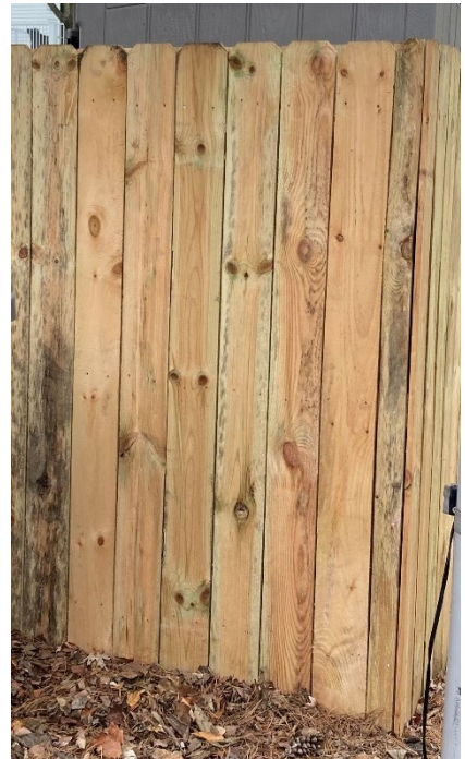
Fence that's been installed
