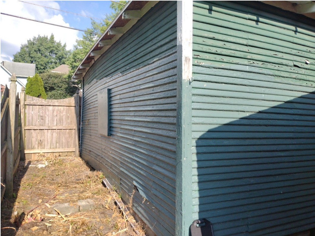
Looking west at south elevation
