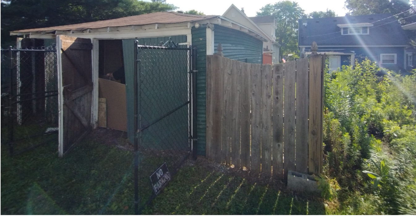
Looking at alley (west) and south elevations
