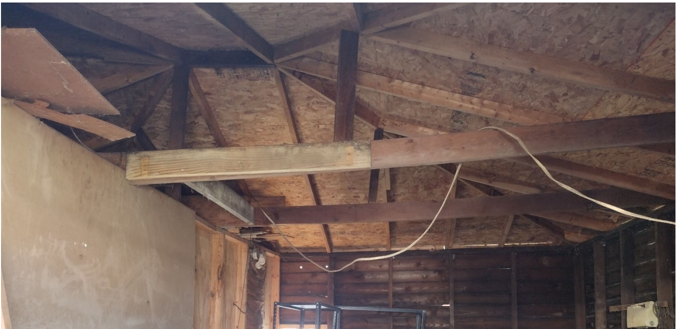
Photo showing previously replaced roof framing and decking
