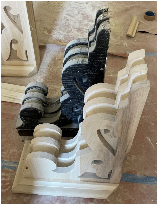
Example of reconstructed corbel in comparison to historic
