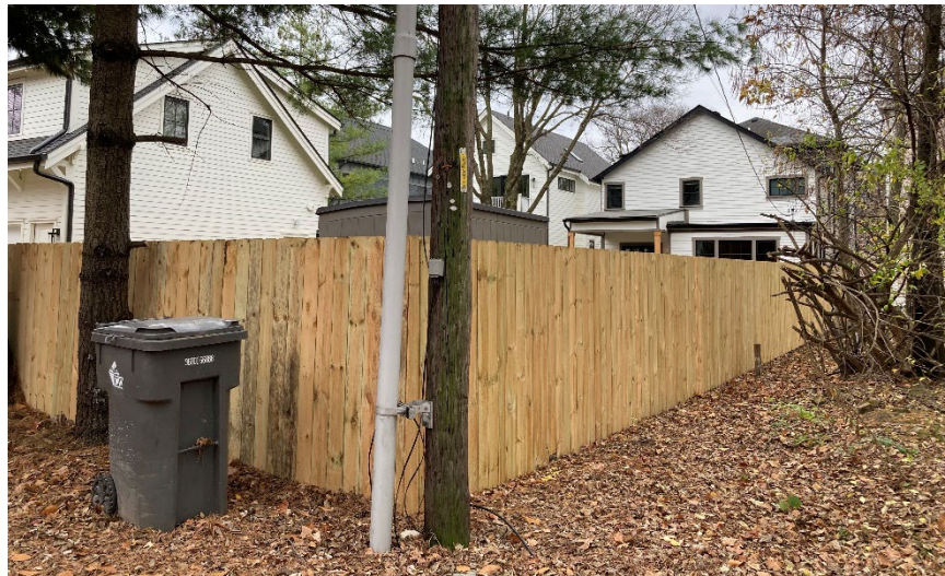
Rear/north side of property (view from alley)
