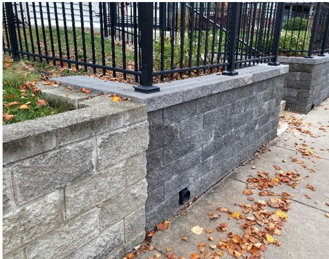
Retaining wall materials (showing neighboring retaining wall to the north)
