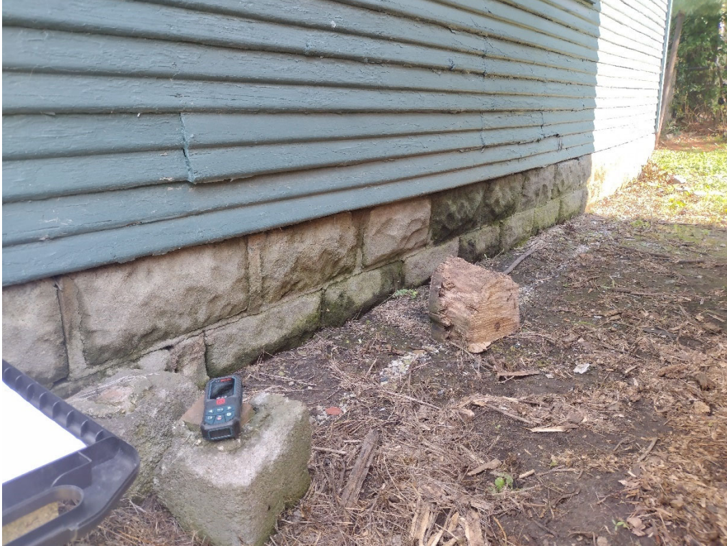
Examples of out of plumb foundation and exterior wall
