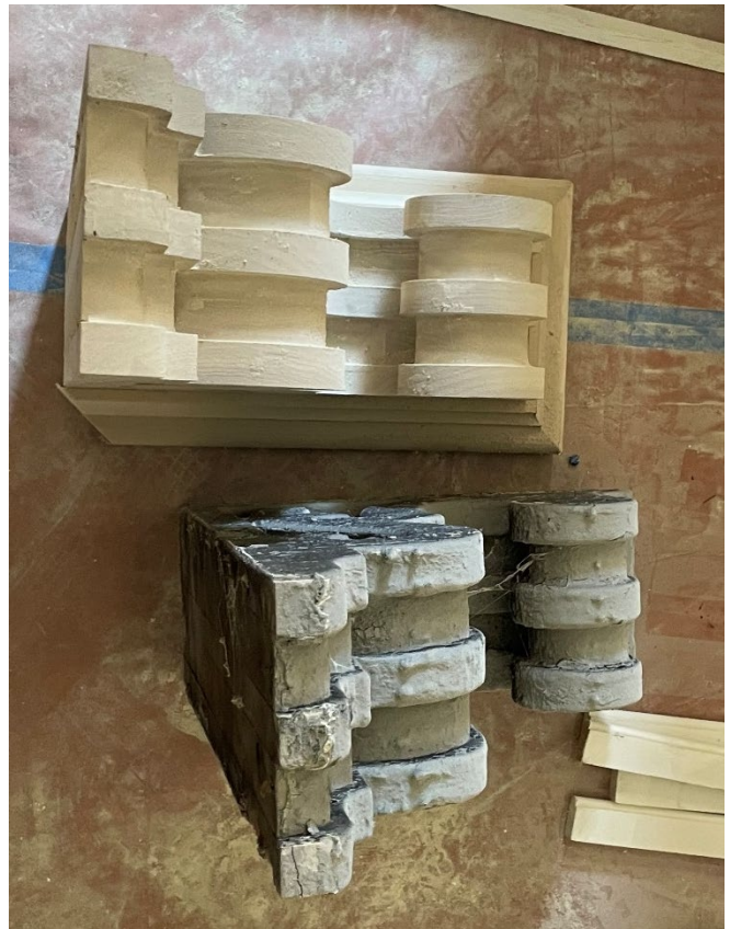
Example of reconstructed corbel in comparison to historic
