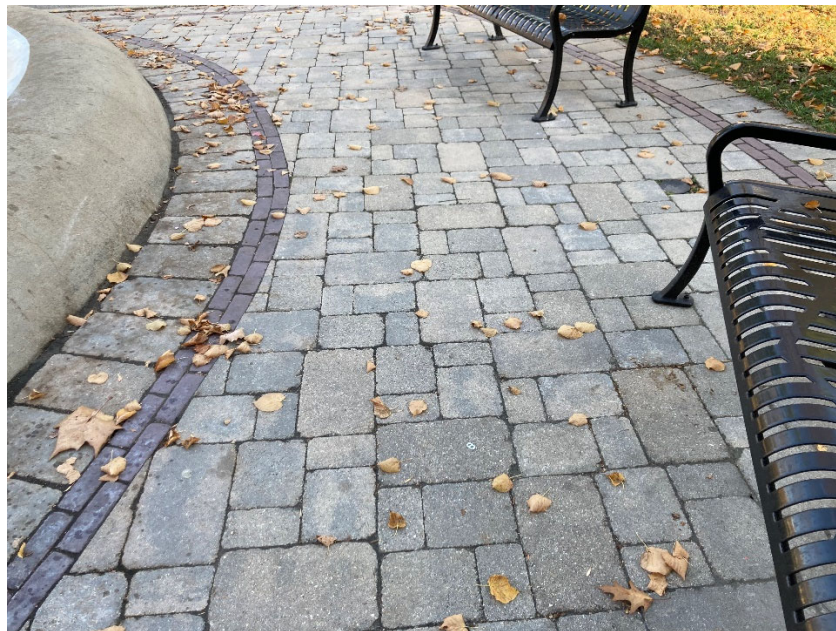
Pavers as installed
