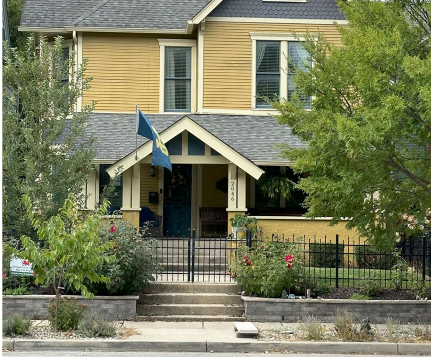
2044 N Alabama (same block, just south) - Retaining wall with front metal fencing.
