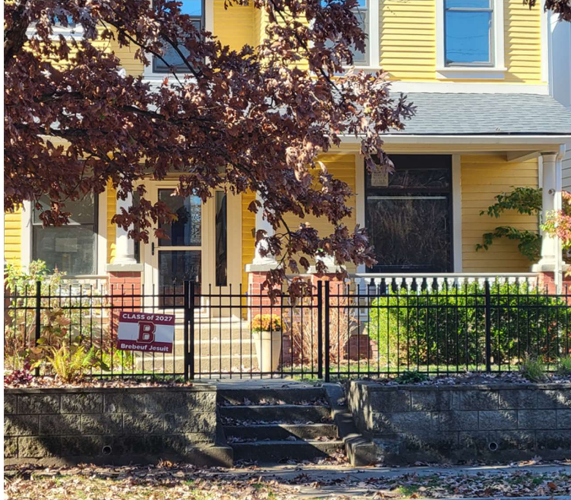
2035 N New Jersey – retaining wall & front metal fencing
