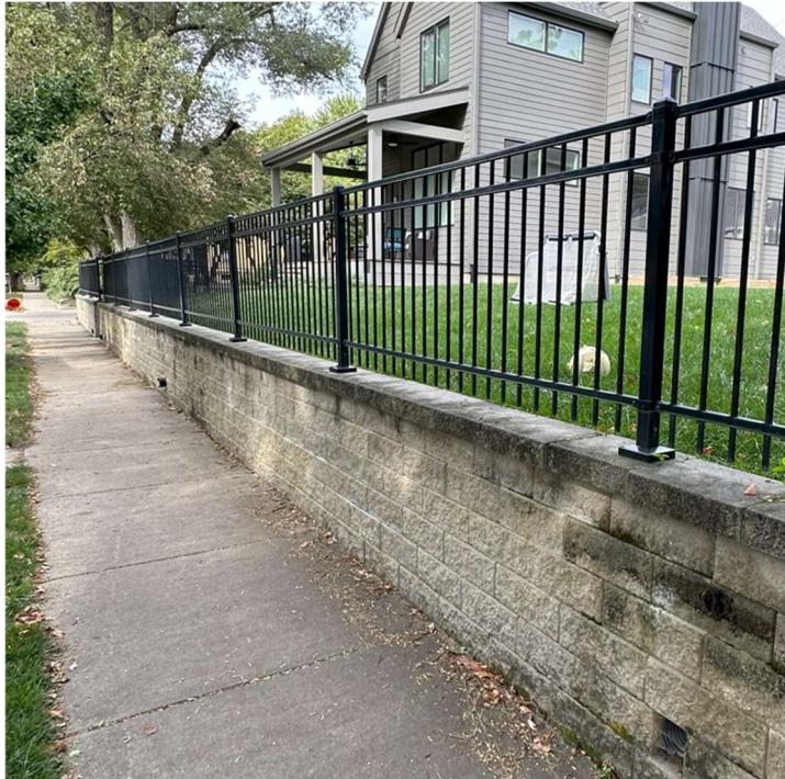
1999 N New Jersey – retaining wall & front metal fence (2 lots total)
