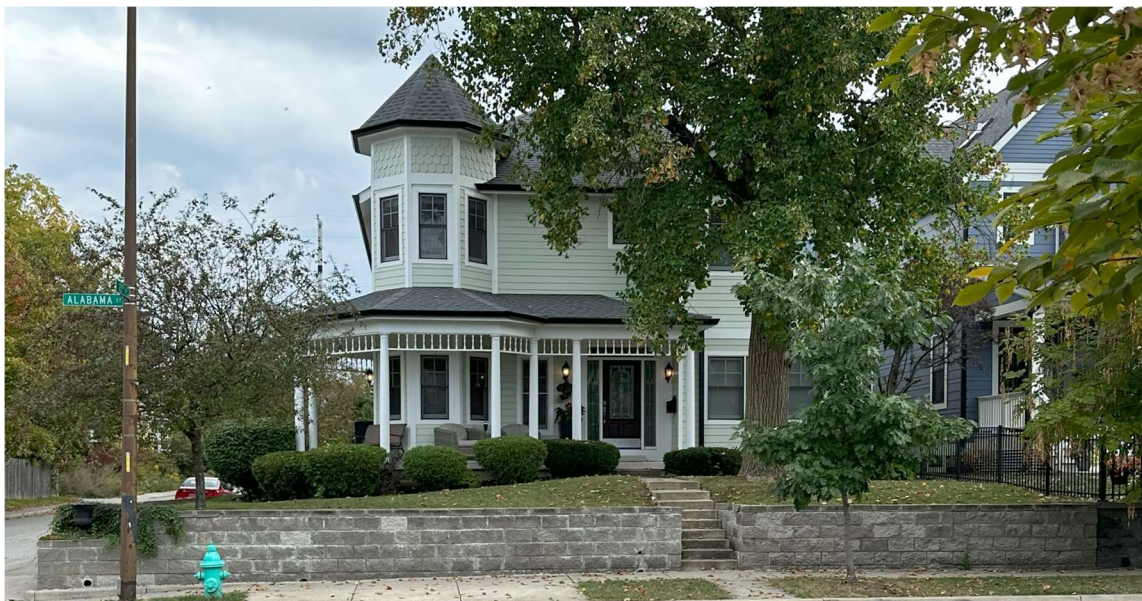
2065 N Alabama (directly north of subject property). Corner of 21 st & Alabama
