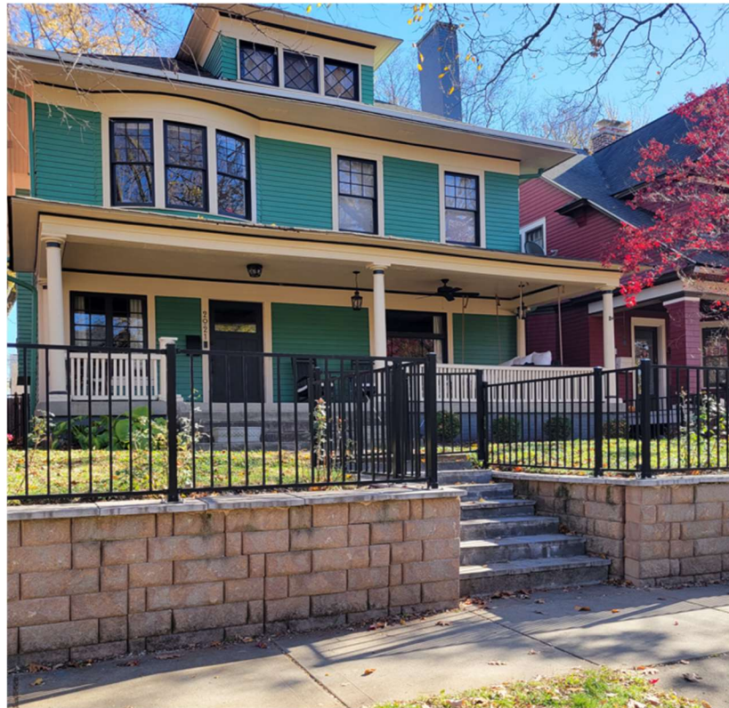
2021 N New Jersey - retaining wall & front metal fencing
