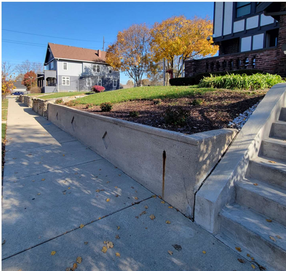
2135 N Alabama Street - historic retaining wall.
