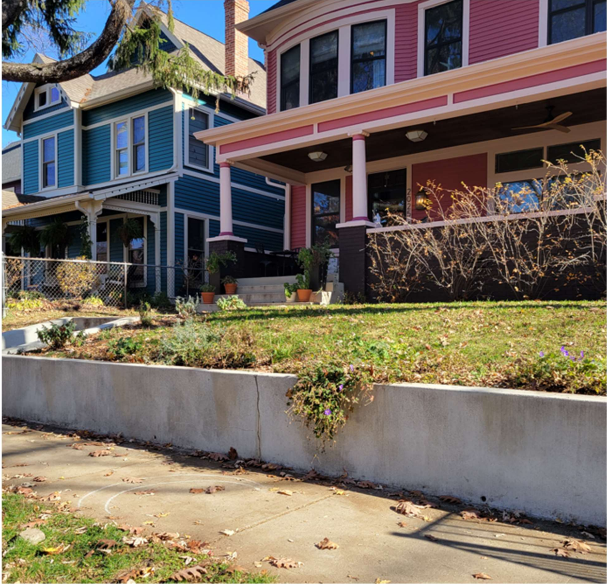
2025 N New Jersey – retaining wall
