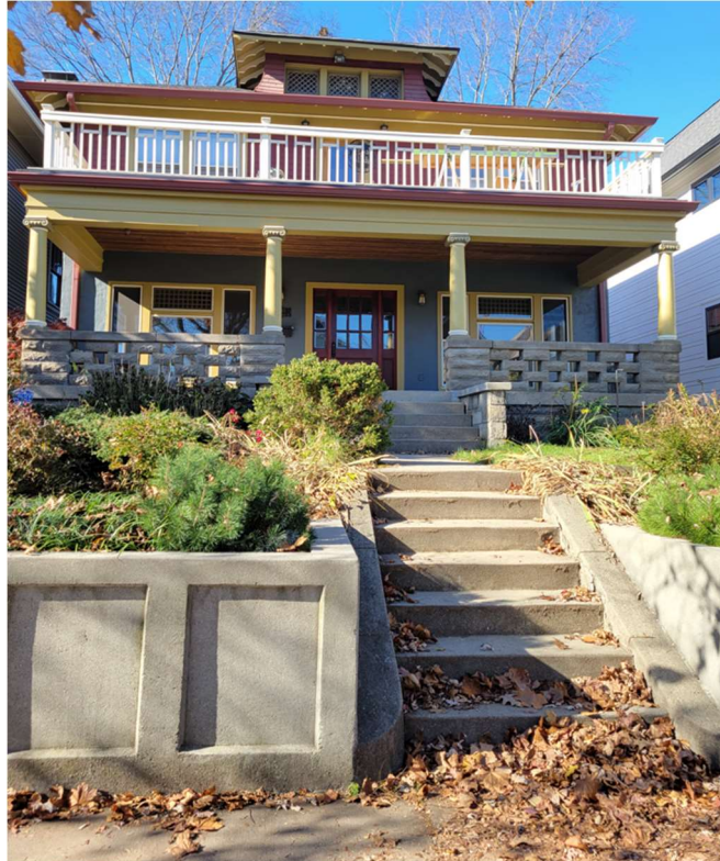
2130 N New Jersey - Retaining wall.
