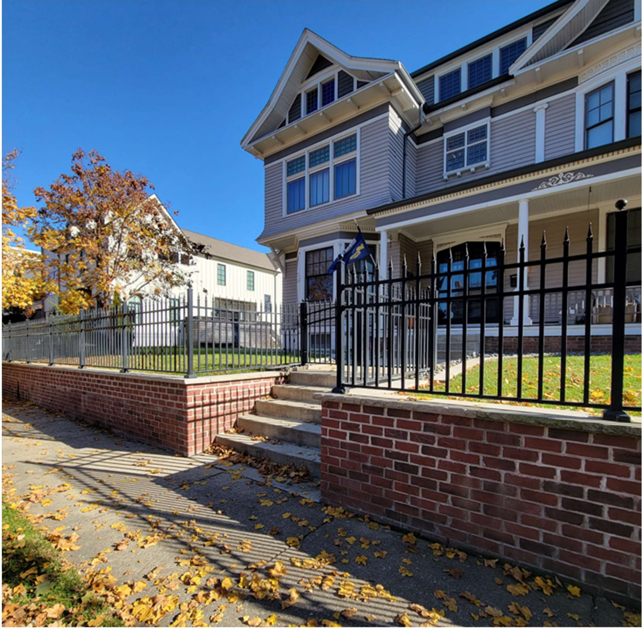
2027 N Delaware Street – 3 lots total - retaining wall & metal fencing
