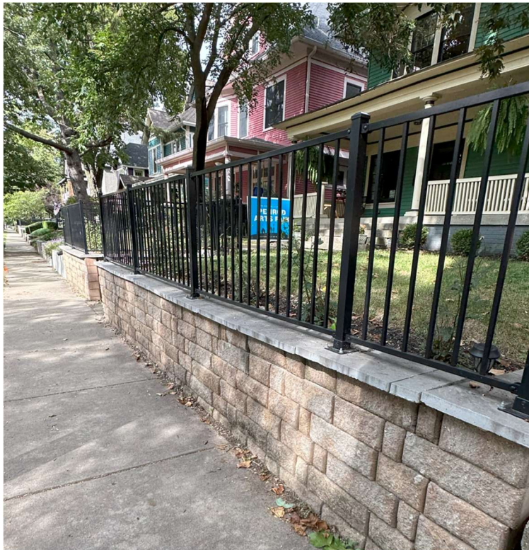
2021 & 2125 N New Jersey – retaining wall & front metal fencing
