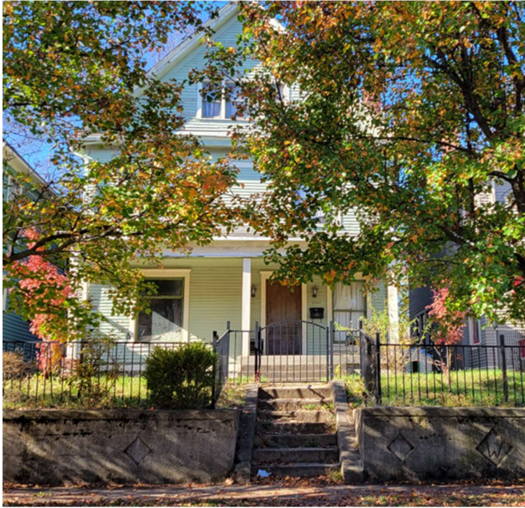
2122 N New Jersey - Retaining wall
