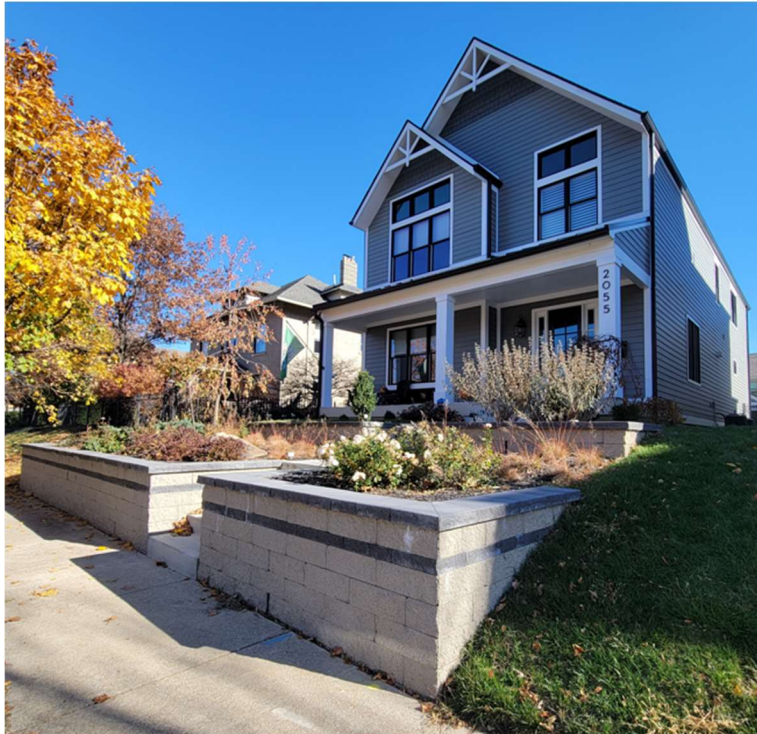
2055 N Delaware St – retaining wall
