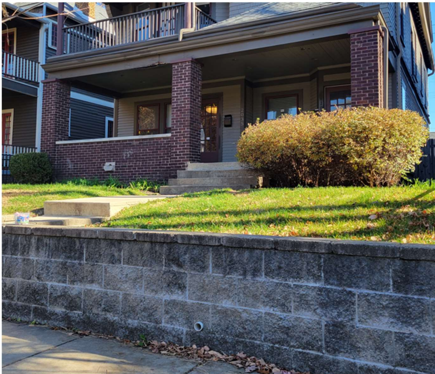
2035 N New Jersey – retaining wall
