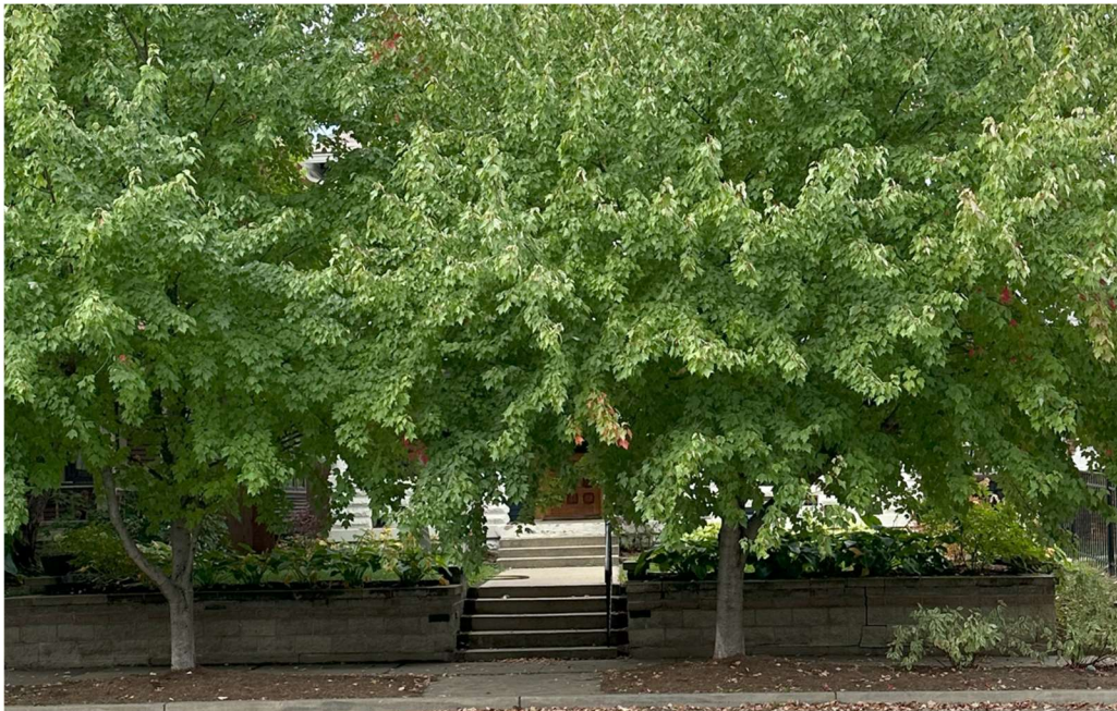
2056 N Alabama (across the street from subject property) – Retaining wall of similar size.
