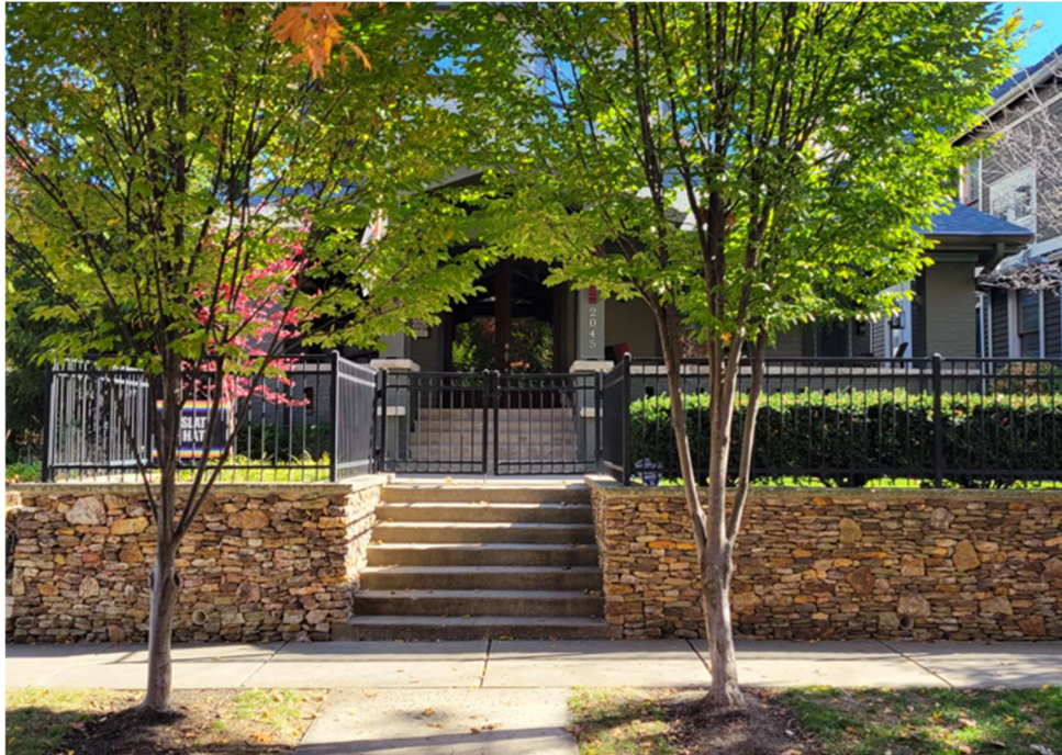
2045 N New Jersey - retaining wall & front metal fencing
