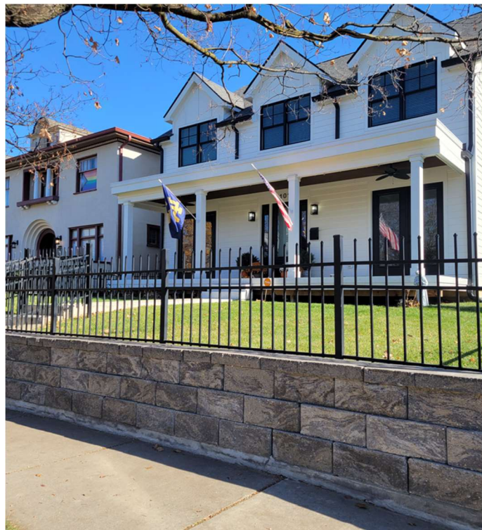
2101 N New Jersey – Retaining wall & front metal fence
