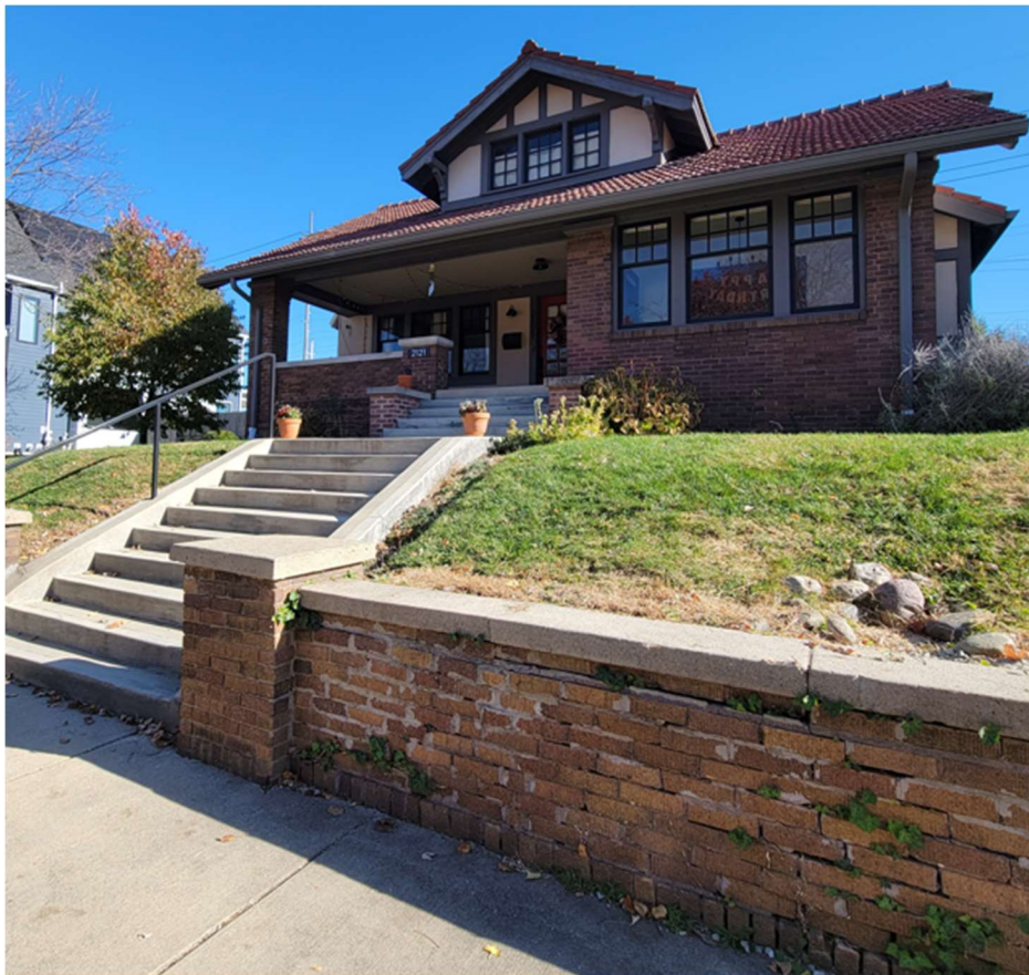
2122 N New Jersey – Retaining wall
