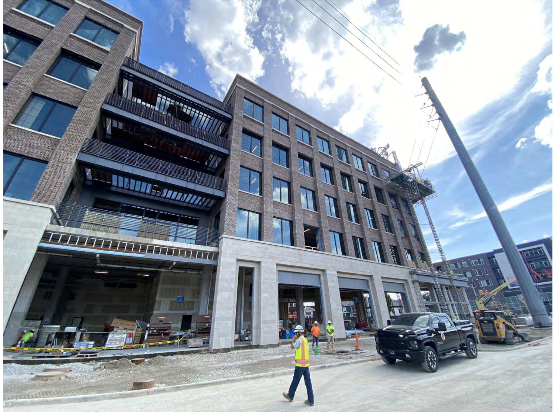
EXISTING STOREFRONT/BALCONIES IN CONSTRUCTION FROM COLLEGE AVE. LOOKING SOUTHEAST
