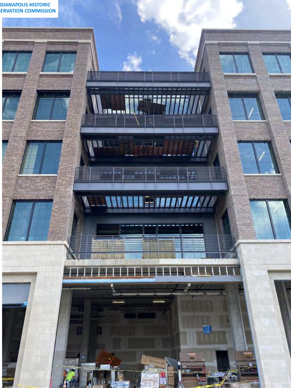
EXISTING STOREFRONT/BALCONIES IN CONSTRUCTION FROM COLLEGE AVE. LOOKING EAST
