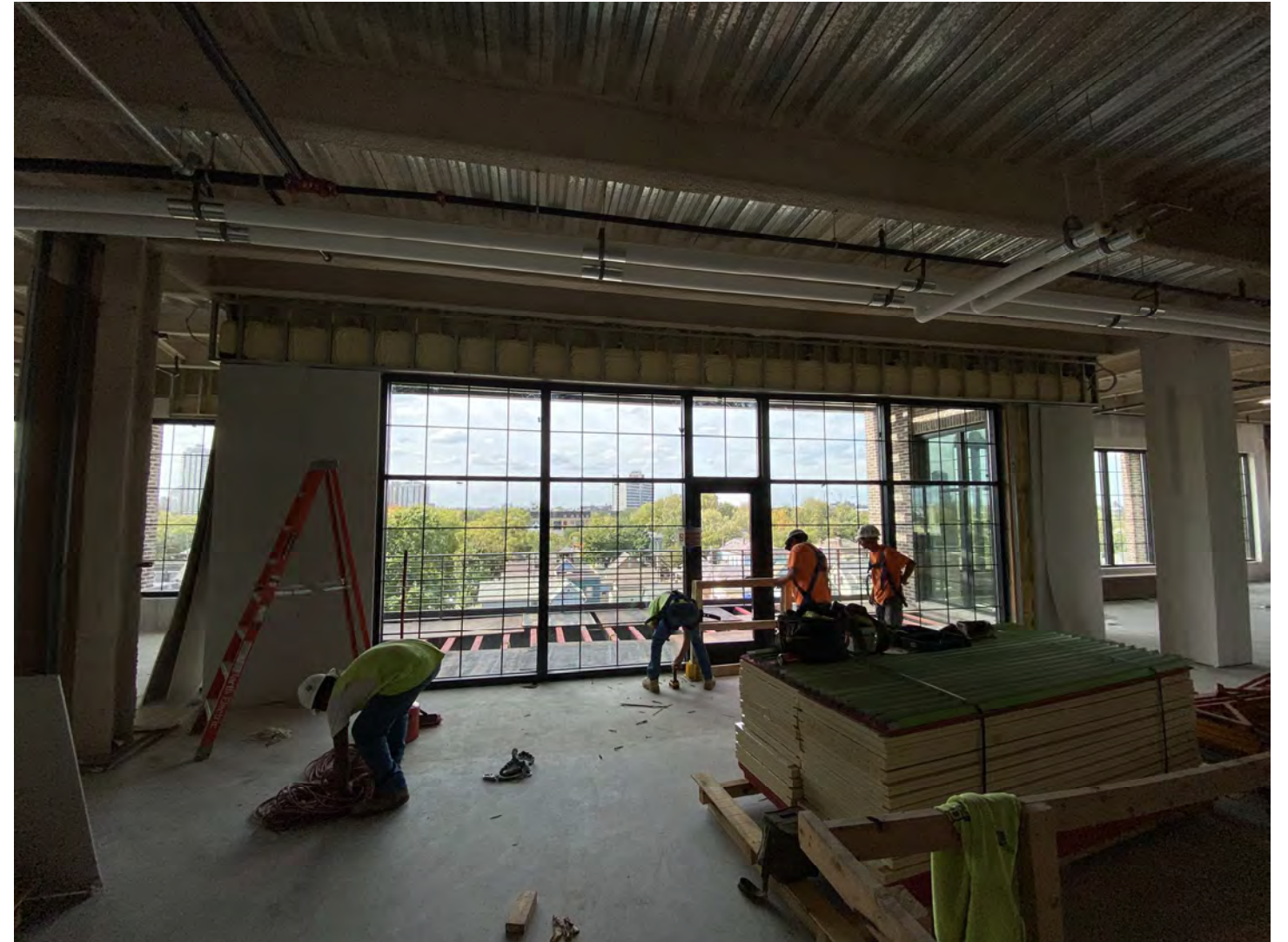
EXISTING STOREFRONT GLAZING FROM INTERIOR
