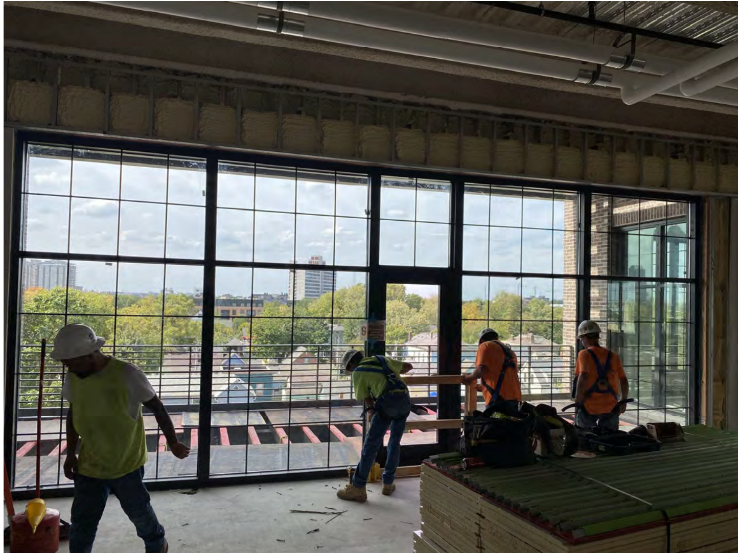
EXISTING STOREFRONT GLAZING FROM INTERIOR
