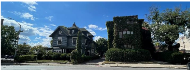
Properties to the south
