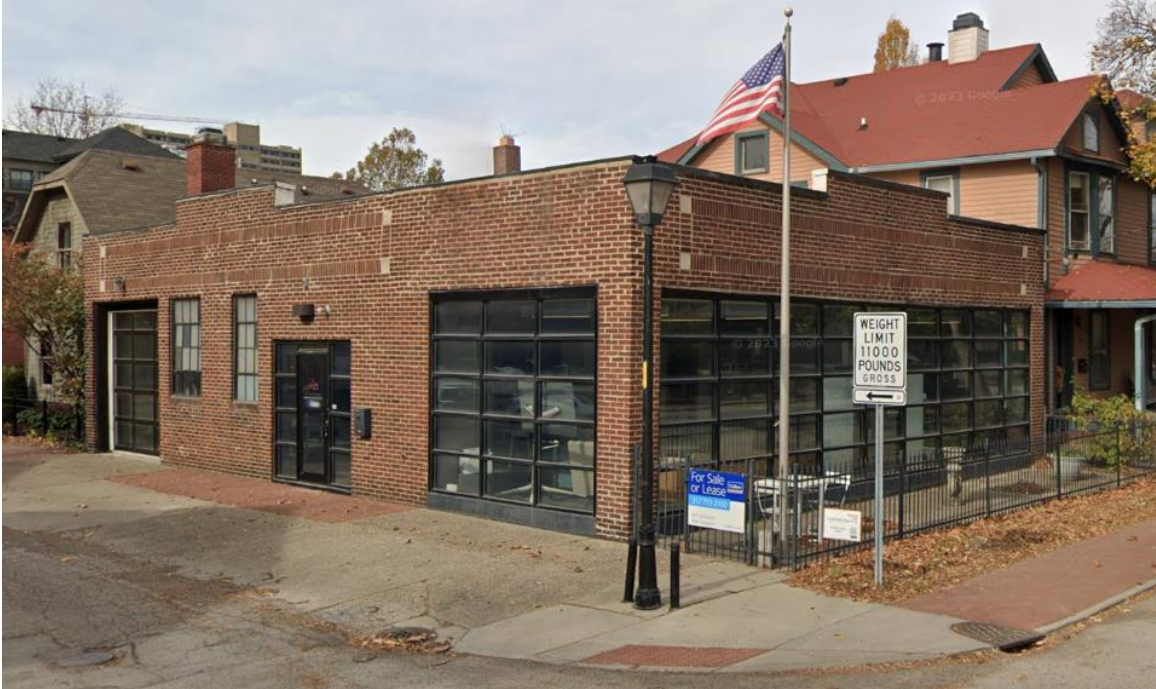
Nov. 2022 Google Street View of front (east) and south elevations
