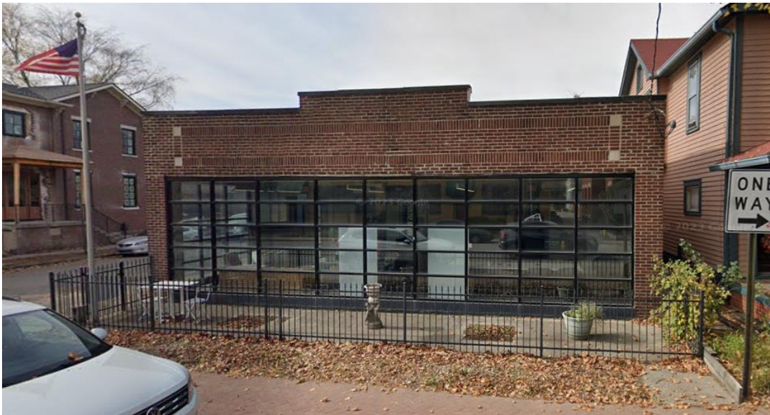
Nov. 2022 Google Street View of front (east) elevation
