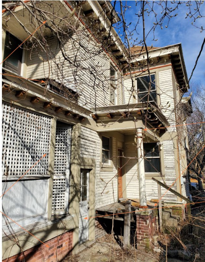
Rear (southwest) corner where a majority of the proposed work is taking place.
