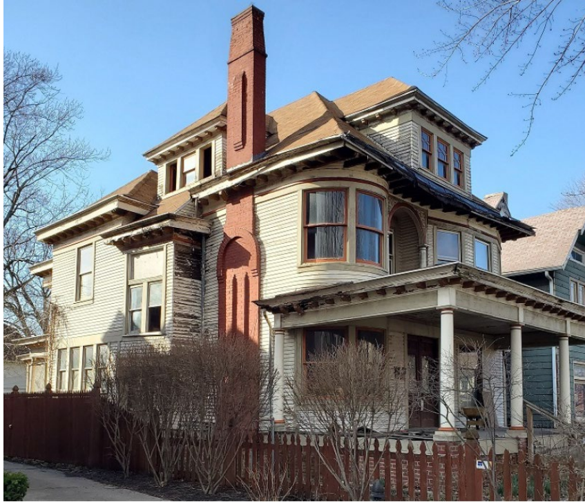
Looking northwest at front (east) and south elevations
