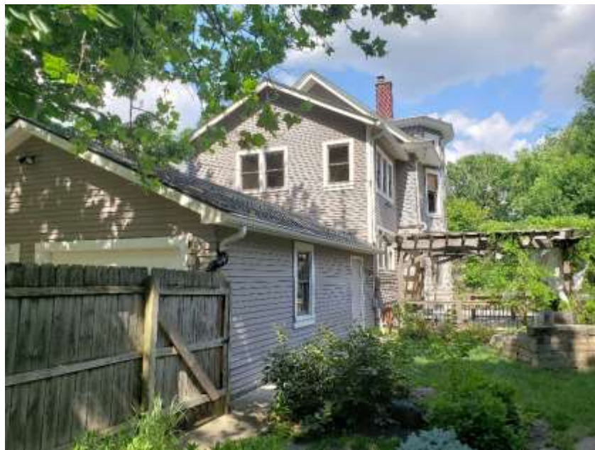
Rear (west) façade of historic house
