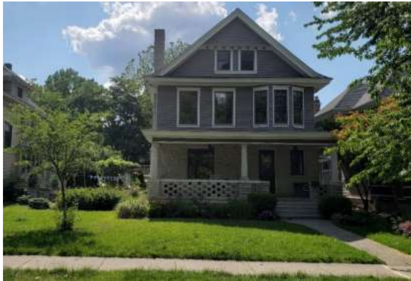
Front (east) façade
