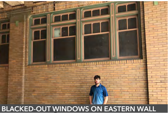
BLACKED-OUT WINDOWS ON EASTERN WALL
