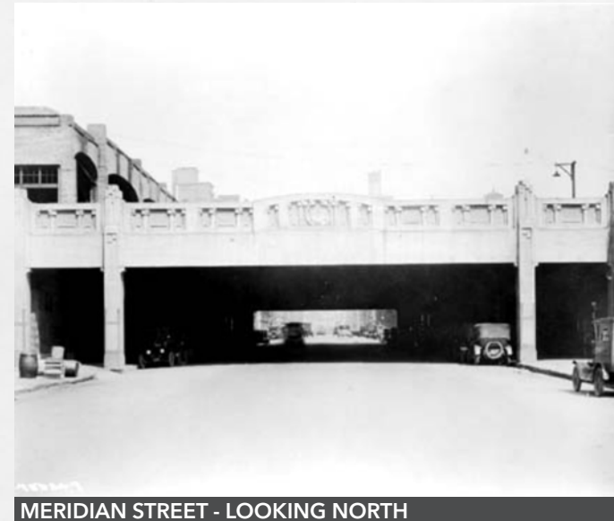
MERIDIAN STREET - LOOKING NORTH
