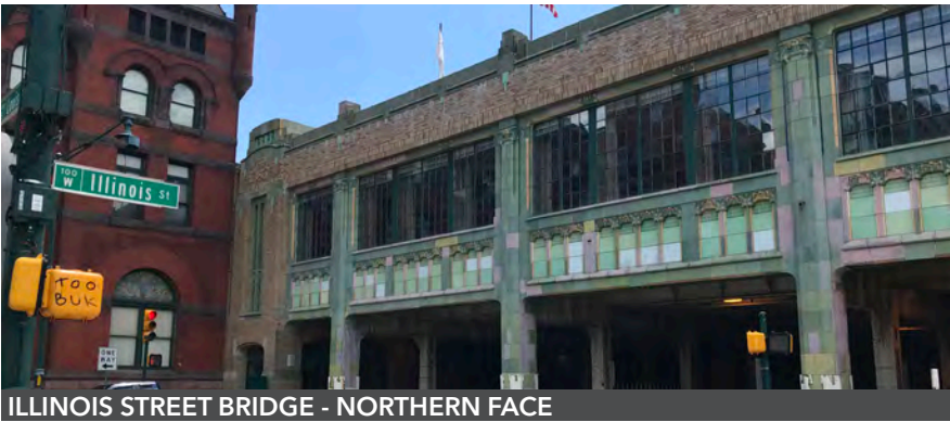
ILLINOIS STREET BRIDGE - NORTHERN FACE
