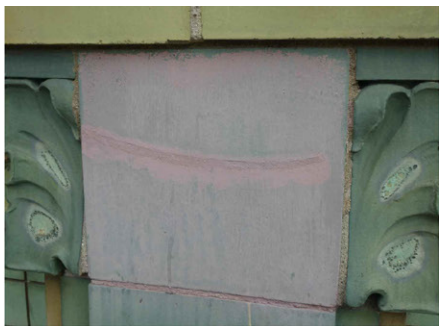
PREVIOUSLY REPAIRED CRACK
