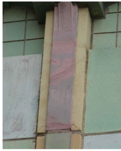
PREVIOUSLY REPAIRED CRACK
