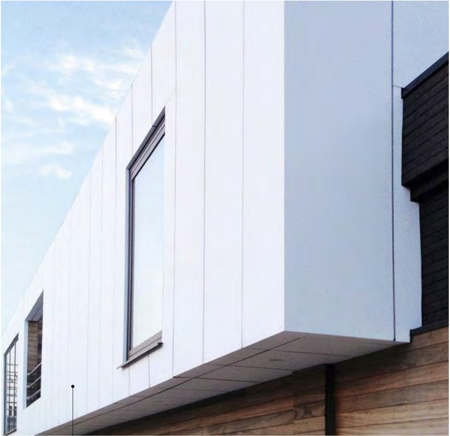
Facade behind the vertical aluminum white fins will be white metal panel, to be surface lit from above and below with continuous RGBW LED lighting.
