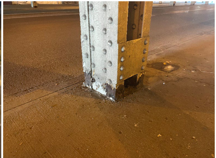
Example of support column conditions under Capitol Avenue bridge
