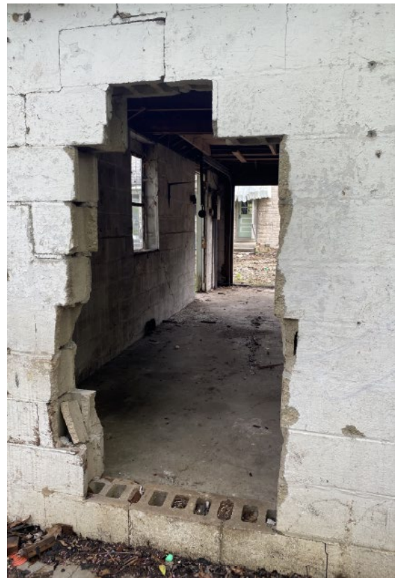
Opening in south exterior block wall of garage. Image on left was taken from inside.
