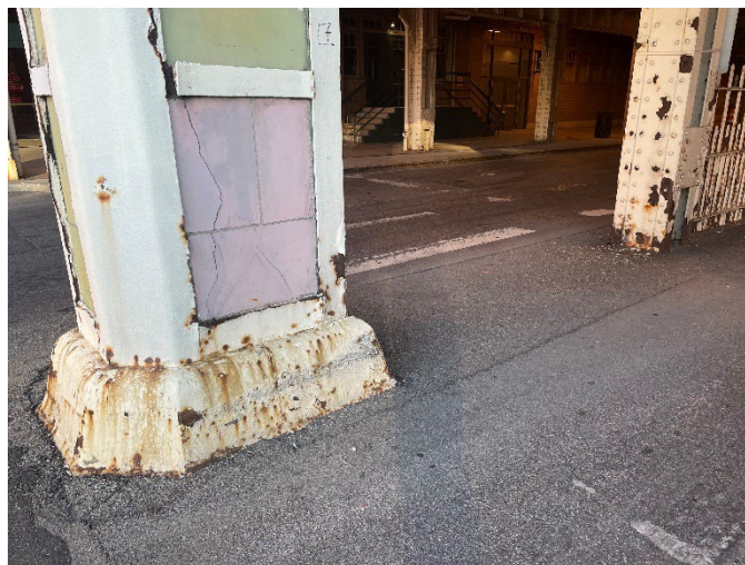
Example of support column conditions under Illinois Street bridge
