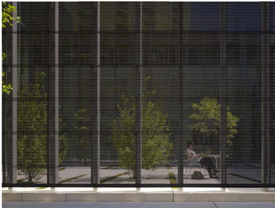
PERFORATED METAL BRISE SOLEIL Inappropriate Materials
