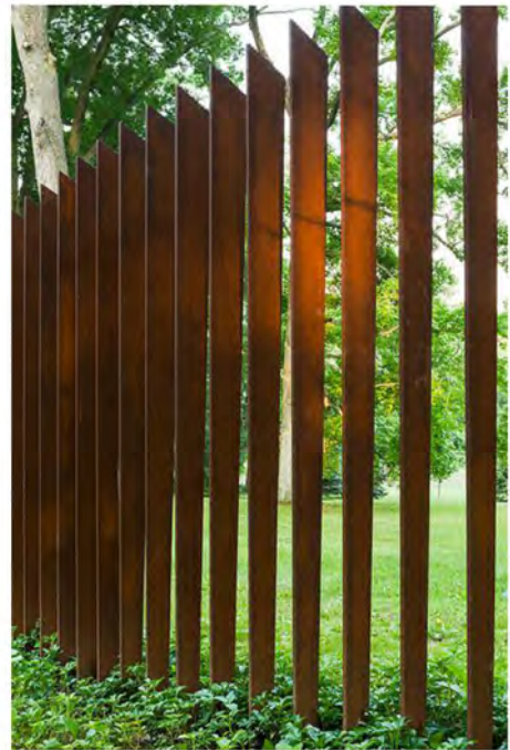
WEATHERED STEEL FENCE Inappropriate Materials
