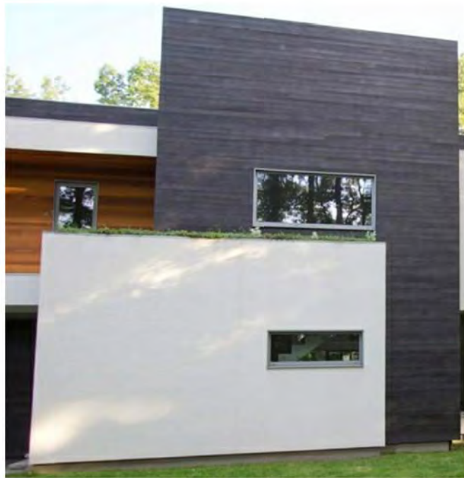
SMOOTH STUCCO Inappropriate Materials
